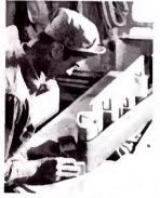
EACH PIECE OF A CROSLEY CABINET is sanded at least five times—first by machine, and finally by hand with a paper so smooth you can't even feel its tiny grains!
