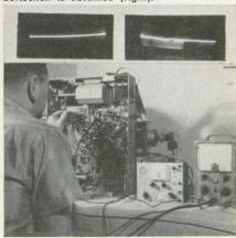
Fig. 9—Injecting Winston's vertical pulse into o IV set's vertical output transformer opens the raster a few inches.
