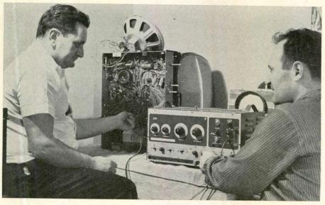
Fig. 6—A shorted grid coupling capacitor was inserted in the vertical output circuit to check vertical problems with each TV sweep circuit instrument.
