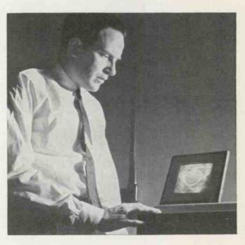
Electronic Panel less than one-half inch thick, invented by Stephen Yando of GT&E Labs., utilizes a new principle to produce a moving, lighted image. In the device shown above, composed of a piezo-electric" ceramic material, a coating of electroluminescent material is actuated by a moving electric charge to produce a luminous display.
