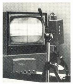
RCA "TV Eye" closed-circuit system is used at Cincinnati Machine Shop of American Can Co. for remote microsccopic inspection of thin scraper blades used in Canco lithography coating presses. Camera projects magnified image of blade on a receiver marked with vertical lines to indicate tolerance limits.
