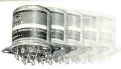
RCA applies manufacturing techniques similar to those used for electron tubes to produce relays for military and commercial applications— 6pdt and 4pdt, rotary solenoid, hermetically sealed, miniaturized, high-speed types featuring welded construction; use af "getter" to absarb organic and metallic vapors far prevention af deterioration of contacts and to insure maximum insulation resistances.
