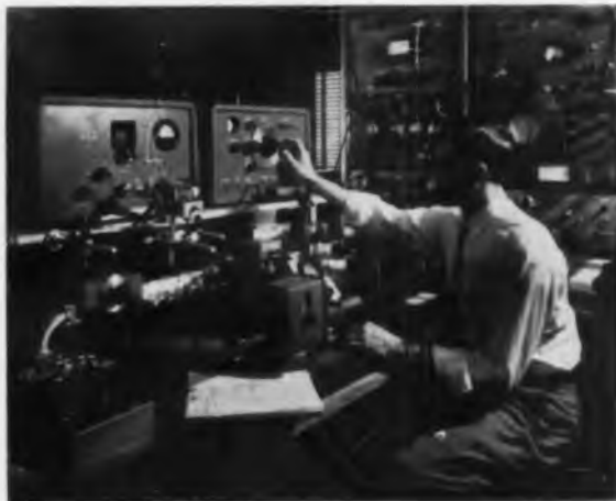
Silicon impurities are determined by electron spin resonance
