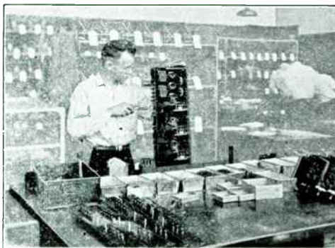
ASSEMBLING THE CHASSIS OF A RADIO RECEIVER
