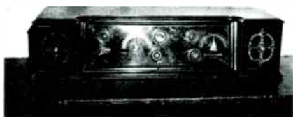
In 1926, the first commercially produced set to operate on AC household current came from Zenith. It freed radio of cumbersome batteries.
