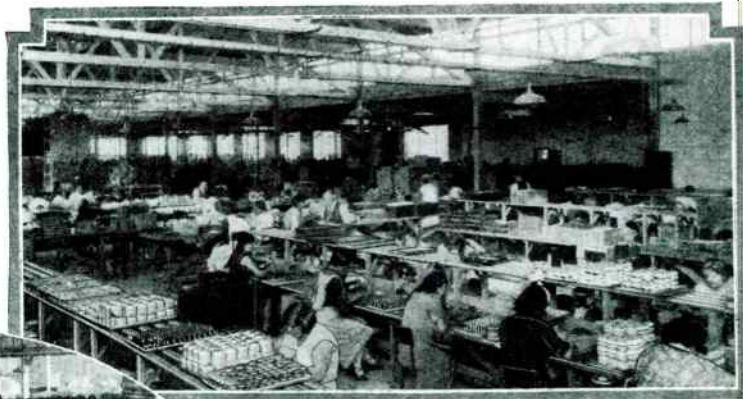
Above, the coil winding department where the enormous number of coils are made that are required daily in the construction of Silver-Marshall Superheterodyne receivers. At the left is the 12,000-foot, centrally located stock room into which all material flows and from which it is drawn as needed by the various departments. All preliminary inspections of raw materials are also made here which greatly speeds up operations in manufacturing departments
