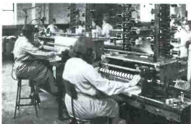
Multiple Coil Winding in the Temple Factory
