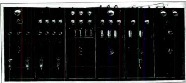
(5000 Watt) Radio Transmitter
