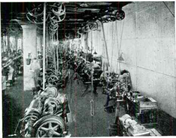
Part of our Automatic Department
