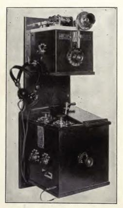
FIGURE 55—Front view of T. Y. K. radiophone transmitter and receiver.
