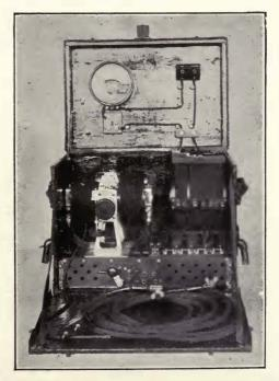
Figure 12—Berliner-Poulsen arc for portable stations.
