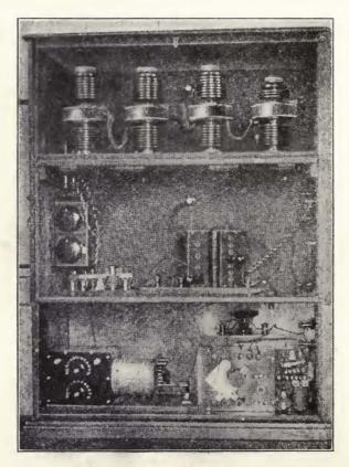
Figure 53—Ditcham radiophone transmitter and receiver.
