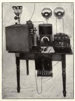
Figure 38—Dubilier radiophone transmitter and receiver.
