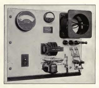
FIGURE 63—de Forest 2 k.w. radiophone panel transmitter.
