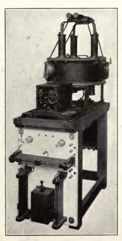
FIGURE 29—Colin and Jeance series enclosed arcs, automatic regulator, and control apparatus.
