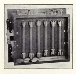
Figure 58—100-to-500-volt direct current coils for direct current supply circuit of T. Y. K. radiophone transmitter.
