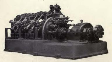
FIGURE 70—Marconi Company "Timed Spark" Discharger.
