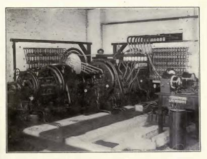
FIGURE 106—Goldschmidt alternator, motor, and reflection circuits at Eilyese, Germany.
