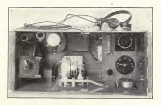
FIGURE 50\*—Aeroplane set with Chaffee gap. Designed by Cutting and Washington.
