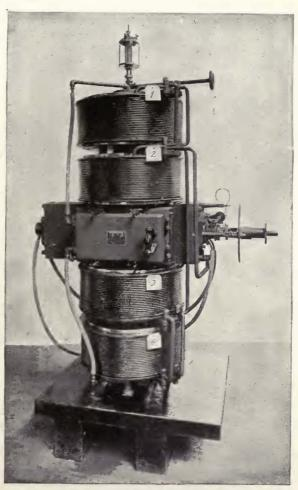
FIGURE 23—Federal Telegraph Company 60 k. w. Poulsen are at Tuckerton.
