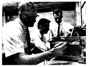
Shown testing the telemetry unit in the IBM lab during an early phase of the Oscar Pulse Code Modulator checkout are (I. to r.) John Champlin, WØZUN, Jeary Vogt, and Don Brouillard. Circuitry in the telemetry unit is built on 20 computer cards. The unit was constructed after working hours during a three-month period.
