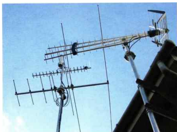
Fig. 4: Kevin Hughes' installation comprising of a compact VF-100 array (HS Publications) for Bands I, II and III plus a separately rotatable PRO-75 u.h.f. array (Televés), with a built-in amplifier.
