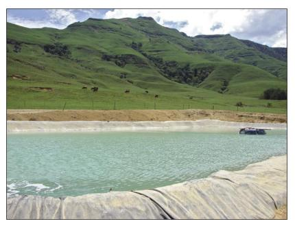
All water from the tunnel is pumped to a holding dam before being treated and released back into the river system. Solid waste is also strictly controlled.
