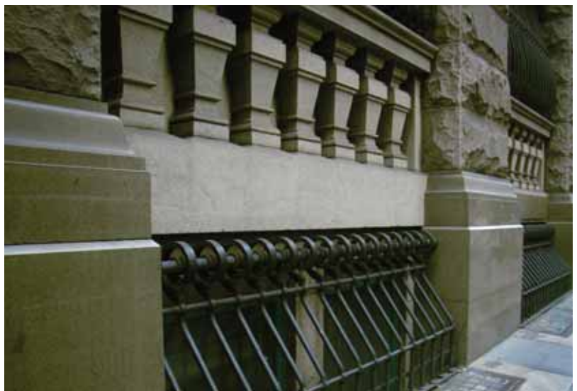
Bowral Trachyte, rough cut, sawn and polished, Angel Place Sydney Photo: J Lemann
