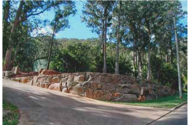
Commemorative Trachyte Entrance Retaining Wall constructed in 2015 with funds raised from sales of the book and a Veolia Mulwara Trust grant. Photo J Lemann
