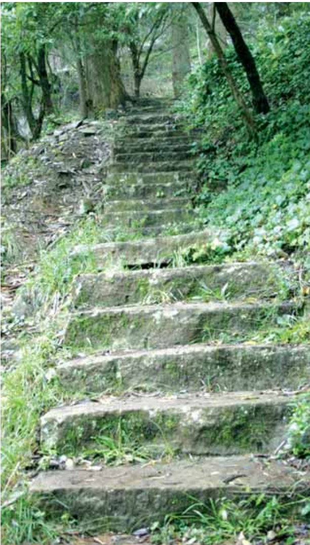
Stone Stairway from Cliff Street Bowral
