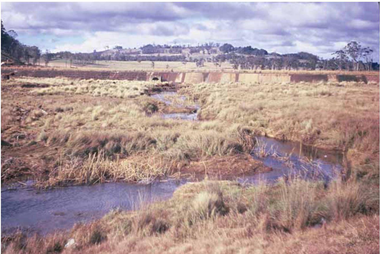
View of the Old Wingecarribee Weir, Sheepwash Road Glenquarry
