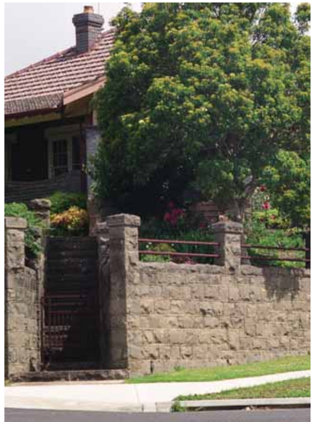
Moss Vale cottage walls
