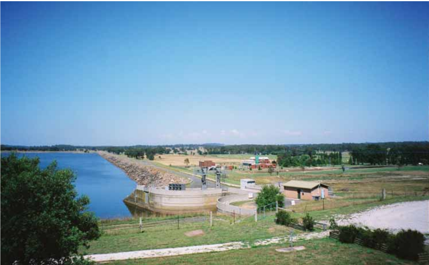
View of the new Wingecarribee Dam and Filtration Plant, Glenquarry
