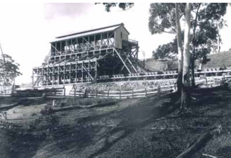
Government ballast crusher
