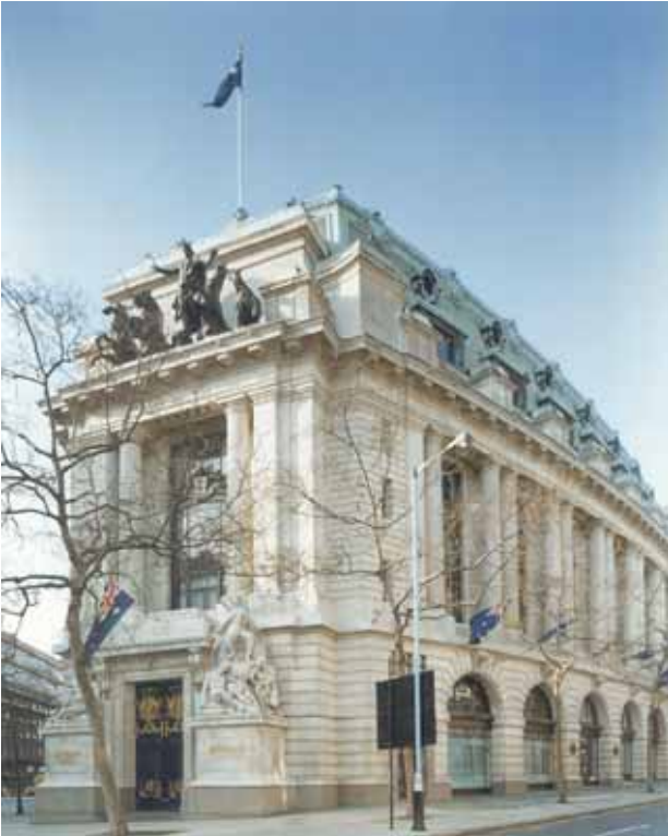
Australia House, London '... a base of Bowral trachyte supports nine stories of yellow sandstone from Bondi quarries - few stones lend themselves to such dignity of treatment as does the deep grey-colour of igneous trachyte of Bowral. Judged whether in the glassy polish of the heavy Tuscan columns at the entrance, or in the chiselled blocks supporting them, its sober hues well accord with the modern classic of the building and the business that it houses...'
