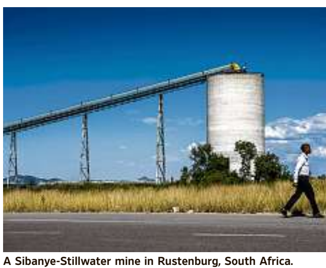
A Sibanye-Stillwater mine in Rustenburg, South Africa.
