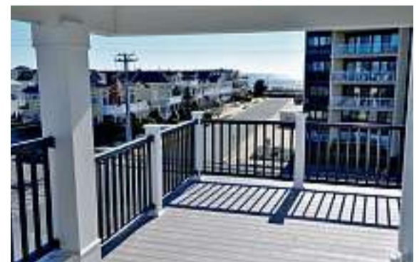
LONGPORT, NJ | $3,695,000 2707 Atlantic Ave 5 BR | 5 FBA, 1 HBA | New Construction Jerome DiPentino 609.432.5588
