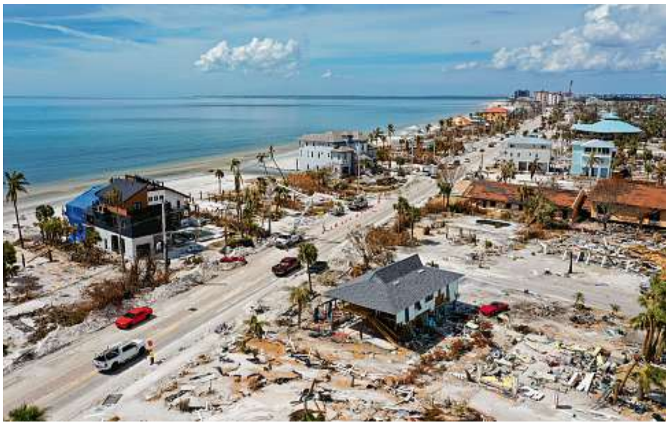
The remnants of Trixie Parkes's home in Fort Myers Beach, Fla., in the aftermath of Hurricane Ian. She plans to sell her property.
