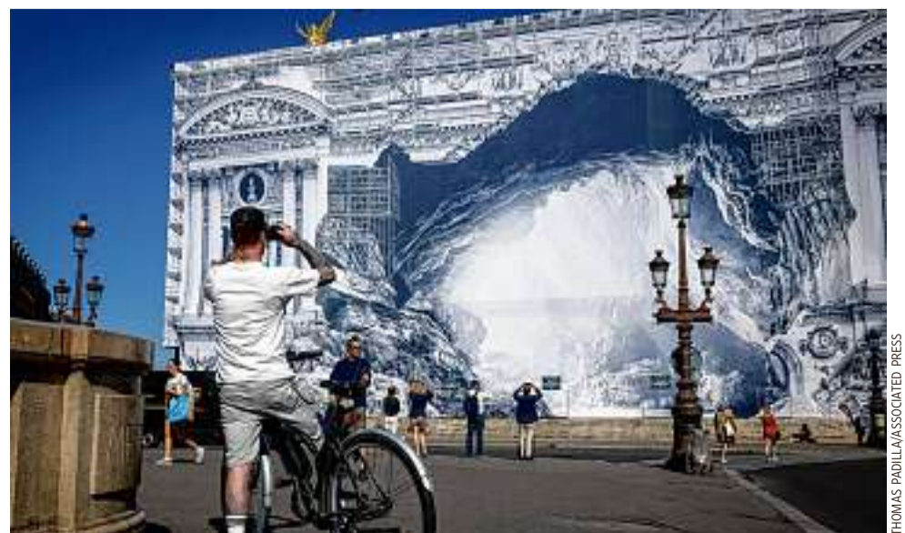
ART SCENE: French street artist JR decorated the facade of the Palais Garnier in Paris with a giant canvas depicting a huge cave. The opera house is under renovation until late 2024.
