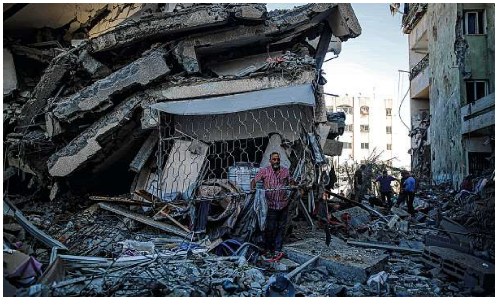
A resident of Gaza City, above, surveys destroyed buildings in the al-Zahra neighborhood. Many won't move from their homes despite the Israeli bombing.
