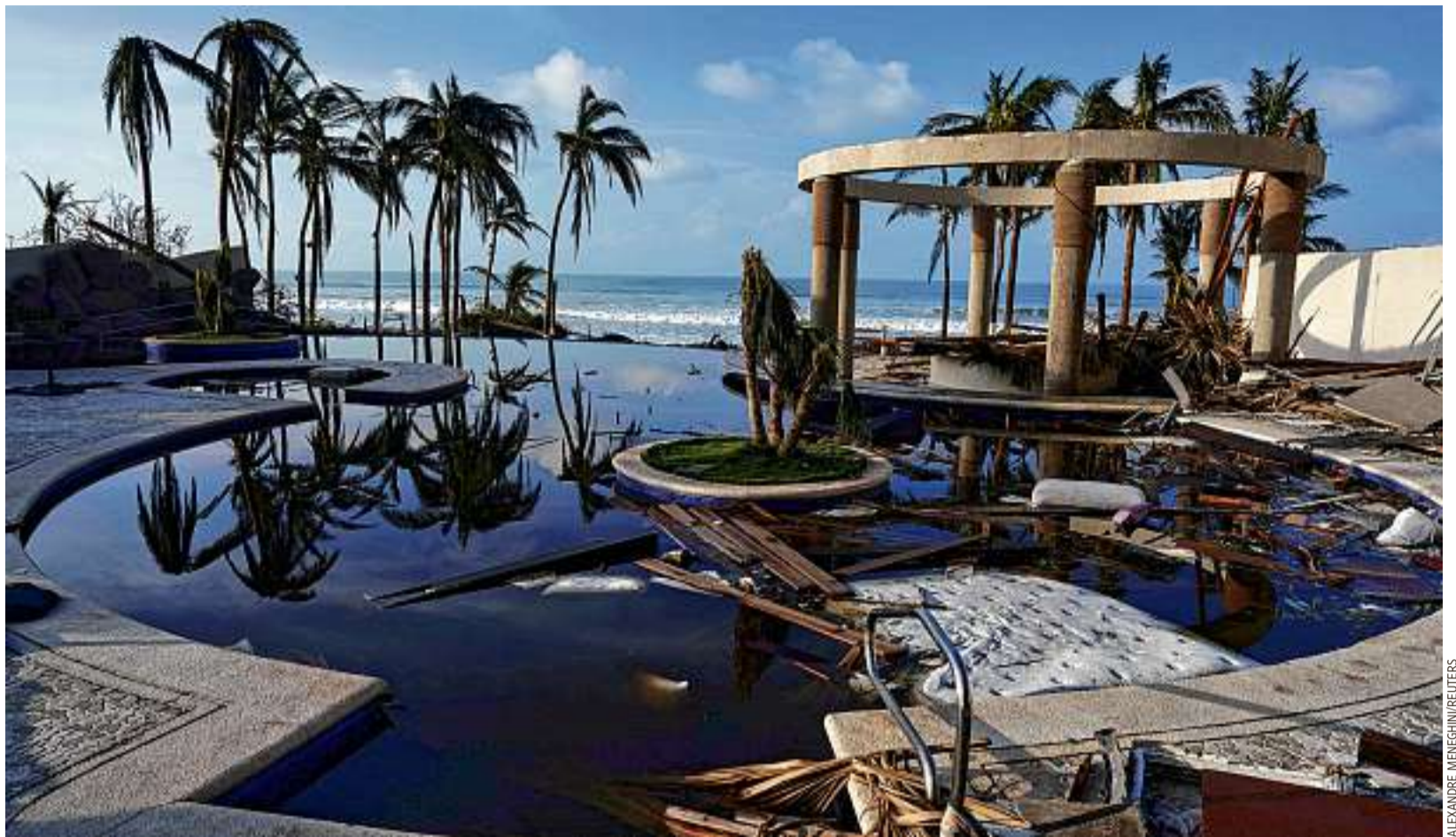
One of many hotels that were damaged when Hurricane Otis hit the resort city of Acapulco, Mexico, after midnight Tuesday, killing at least 27 people.
