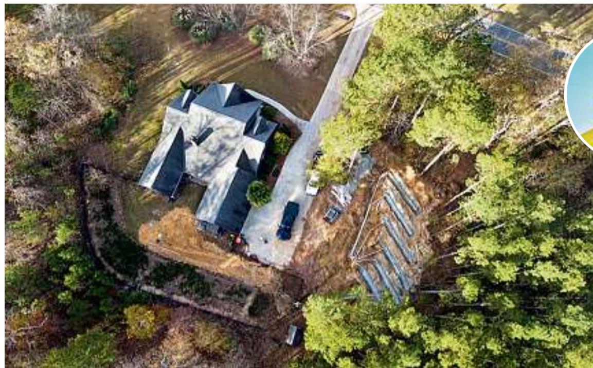
Aerial view of a septic system installation with leach field (right).
