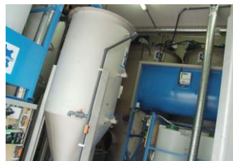
Figure 2 UASB in Sneek where source separated BW is treated in a decentralized approach
