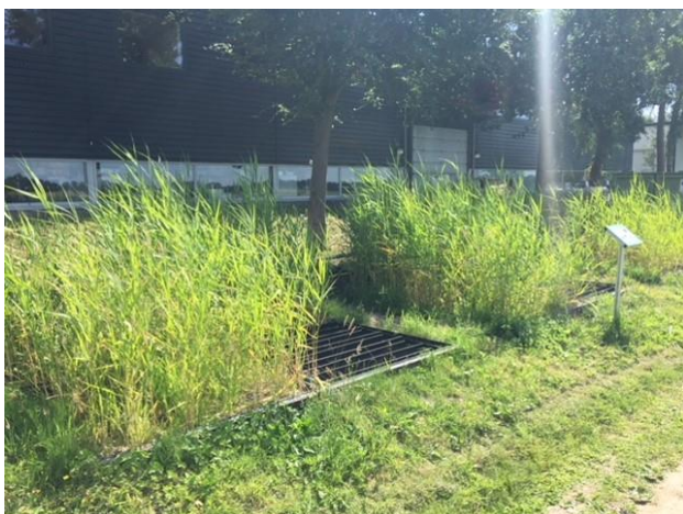
Figure 1. Pilot-scale constructed wetlands next to the laboratories of ETE.
