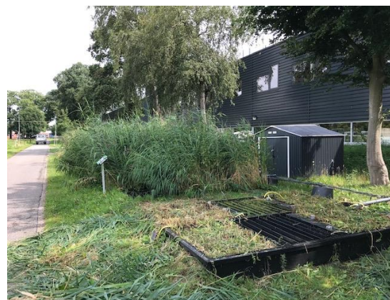
Figure 2. The removal of the vegetation from the pilot-scale constructed wetlands in summer.
