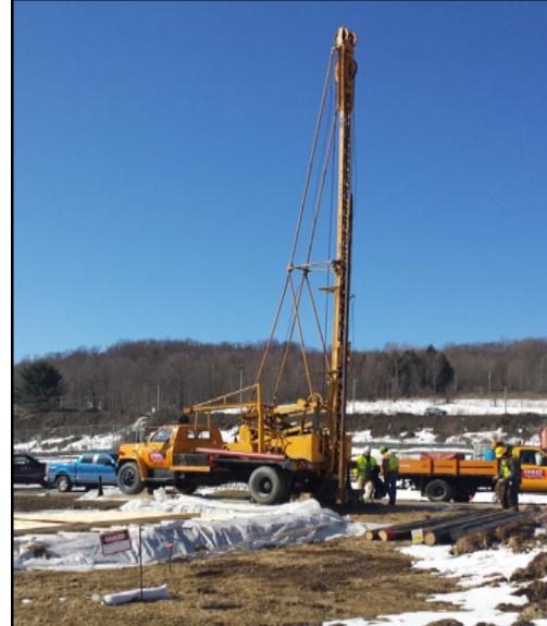
Installation of Groundwater Supply Wells
