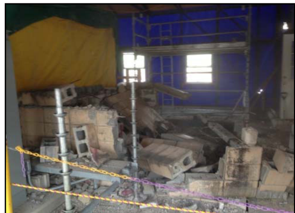
Con-Ed Building Demolition
