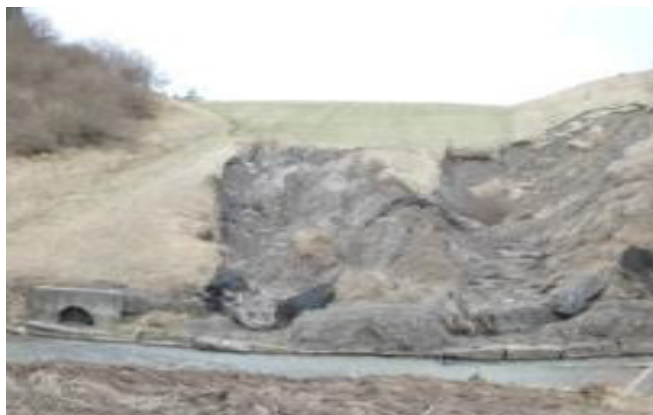
Lake 1 Spillway before 2014 Repairs
