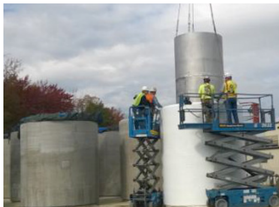
Loading Overpack into a Cask
