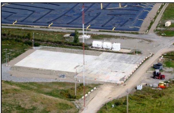
HLW Cask Storage Pad
