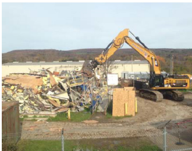
Demolition of the Environmental Lab
