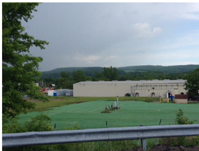
Restoration of Environmental Lab area
