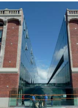
The «Sugar warehouse» in Dunkerque (59) Pierre-Louis Faloci Architect
