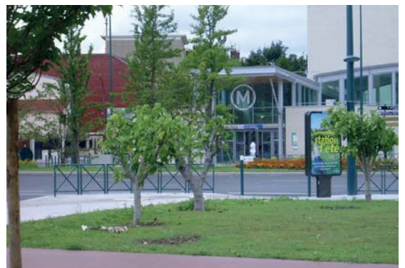
Laying out of a secondary highway road in Asnières and Gennevilliers (92) TGT Architect - Acte 2 Paysage Landscape Architect
