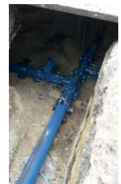
SEDIF - Drinking waterworks renewal in the south of the Paris region (91, 92, 94)
