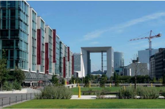
Terraces in Seine Arches Area urban Planning for EPADESA in Nanterre (92) TGT Architect and Planner
