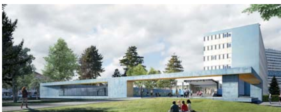
Animal Housing Facility at Mondor Institute for Biomedical Research In Paris Créteil University (94) - Celnickier & Grabli Architect
