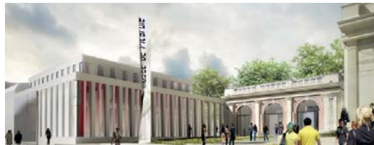
Refurbishment of the Museum of Picardie in Amiens (80) Frenak & Jullien Architect
