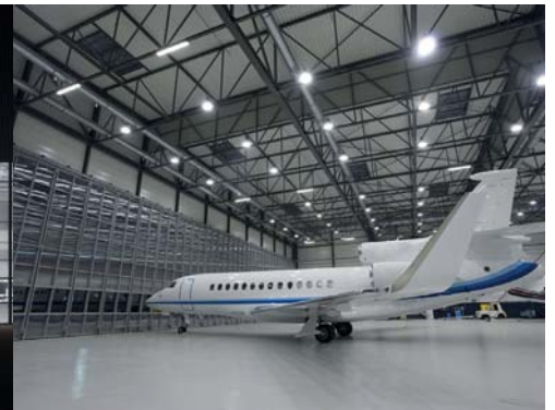
Dassault Falcon 7X maintenance Hanger in Le Bourget Airport (93) Christian Devilliers Architect
