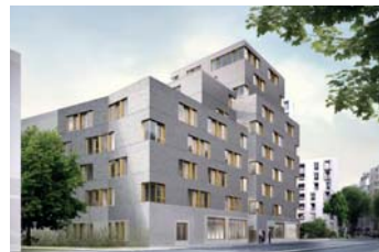
Student housing for RIVP in Paris (75) Nicolas Reymond Architect
