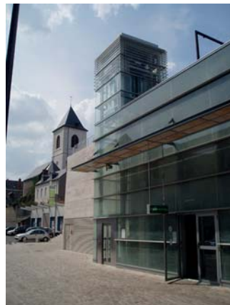
Public car park in Orléans (45) Atelier Tudelle Architect
