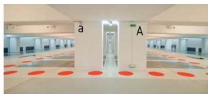
Restructuration of underground car-Park in Nanterre (92) - TGT Architect
