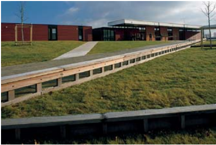
Beach and Swimming Area in the public regional leisure centre in Torcy (77) Michel Rémon – Jacques Coulon Architects
