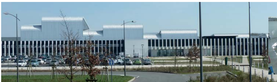
IndustriLab, aeronautic technology transfer centre specialized in robotics and composite materials in Méaulte (60) Michel Rémon Architect
