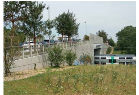
Bridge over RER A in Champs-sur-Marne (77) Ateliers Lion Architect
