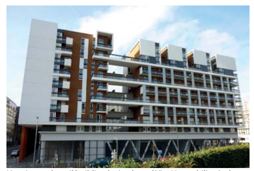
Housing and retail building by Icade and Vinci Immobilier Arche en Seine in Nanterre (92) - Ateliers 234 Architect
