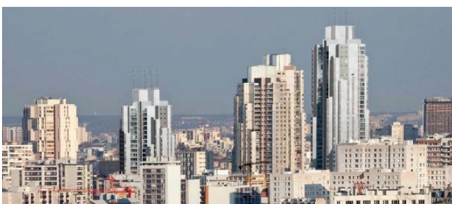
Refurbishment of «Prélude and Sonate» Towers for Immobilière 3F in Paris (75) Ateliers Lion Architect
