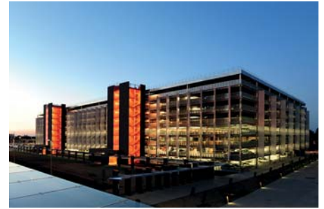
Above-ground parking structure (3,200 lots) in Toulouse-Blagnac (31) SCAU Azema Architects
