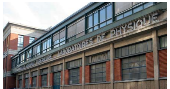
Refurbishment of Physics, Chemistry and Environmental studies laboratories in Paris (75) PHD Architect - IGREC INGENIERIE Project Manager and Representative
