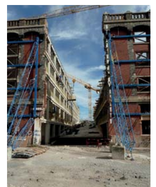
The «Sugar warehouse» in Dunkerque (59) - Pierre-Louis FALOCI Architect
