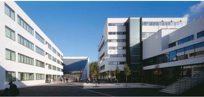
Paris XII University - Law faculty and library in Creteil (94) Michel Rémon Architect
