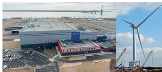
Offshore assembly wind power plant in Montoir de Bretagne (44) Philippe Cointet Architect - Quille Company- EGIS Grand Ouest
