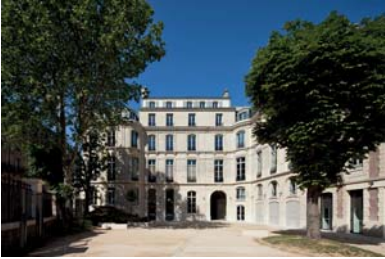
Refurbishment of Wendel Mansion into an elementary school in Paris (75) - SCAU Architect
