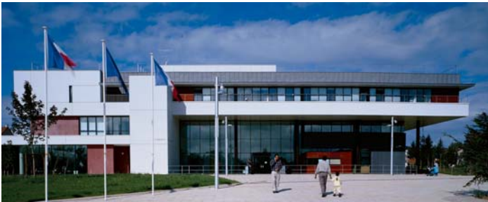
Regional Administrative Centre in Sarcelles (95) for the French Home Office Michel Rémon Architect
