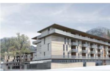
Aegide Senior Residence in Briançon (05) Pierre-Louis Faloci Architect
