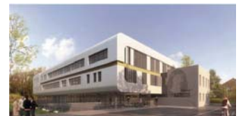
Incubator for innovative enterprises in Cite Descartes à Champs sur Marne (77) Studio Bellecour Architect
