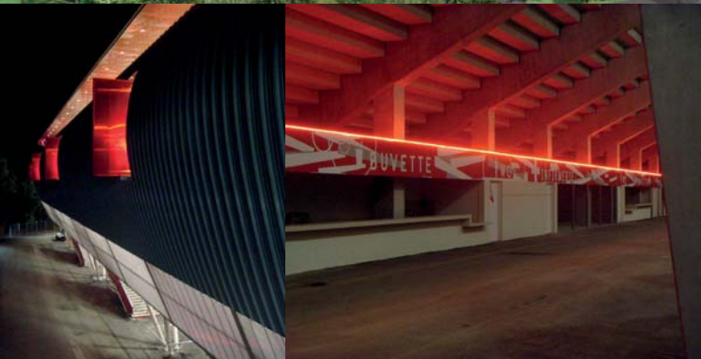
Re-structuring and refurbishment of Gaston Gérard Stadium in Dijon (21) Michel Rémon Architect
