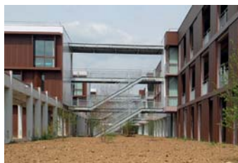
Farming vocational High School in Brie Comte Robert (77) - Ateliers 234 Architect
