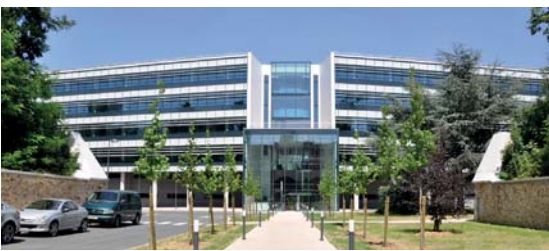
Office and research building for ONERA National Office for Aerospace Studies and Research in Palaiseau (91) - ABH Architect
