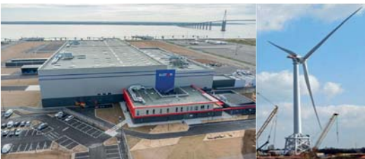
Offshore assembly wind power plant in Montoir de Bretagne (44) Philippe Cointet Architect - Quille Company- EGIS Grand Ouest
