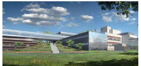
Construction of the Institute of integrative Biology of the Cell in Gif-sur-Yvette (91) - N. Ragueneau & A. Roux - Michel Rémon Architects
