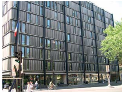
House of Human Sciences in Paris (75) François Chatillon, ACMH - Michel Rémon Architects
