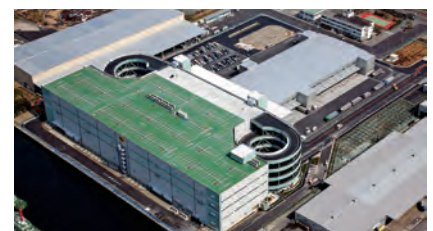
10—Aerial view of Yamato Transport's Kanagawa Logistics Terminal completed in 2007. At the time, it was the Yamato Group's first full-scale logistics terminal, including a logistics building that housed the Kanagawa Sorting Hub and Yamato Logistics.
