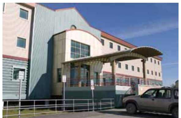
Community Health Services Building, YKHC Corporate Headquarters.
