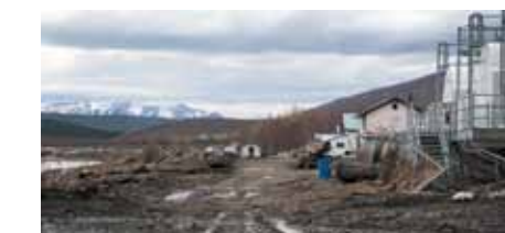
Flood damage at Crooked Creek.
