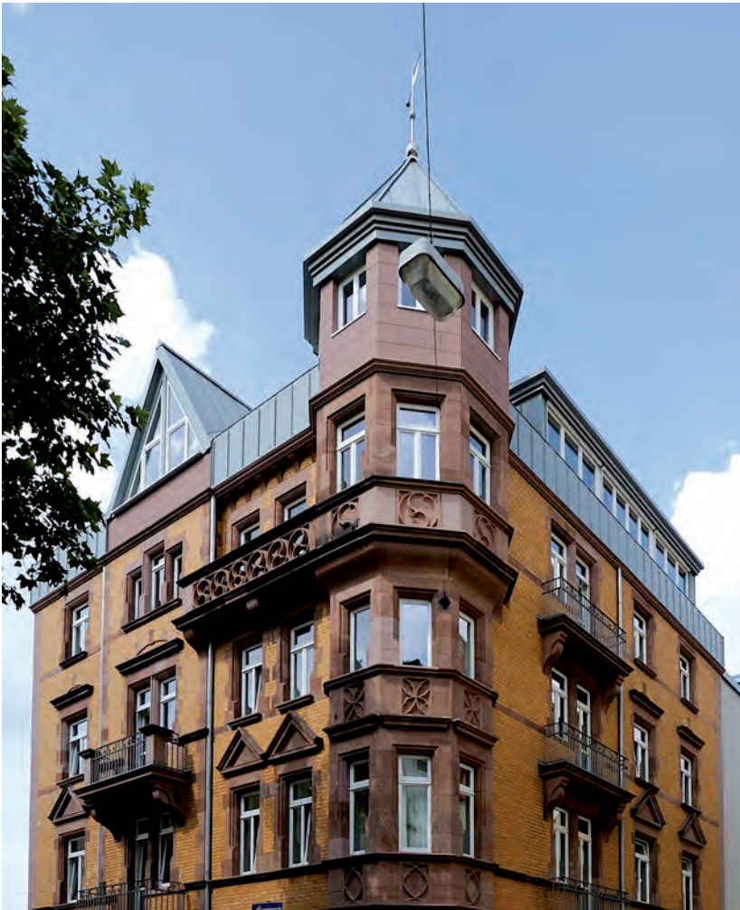
The Addiction Center with the historic facade in J 4.
