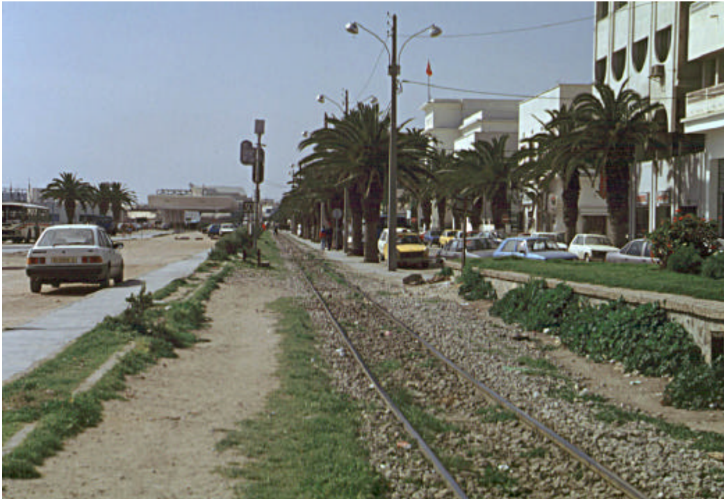
Fig. 21: Railway tracks in the modern town near the harbour.
