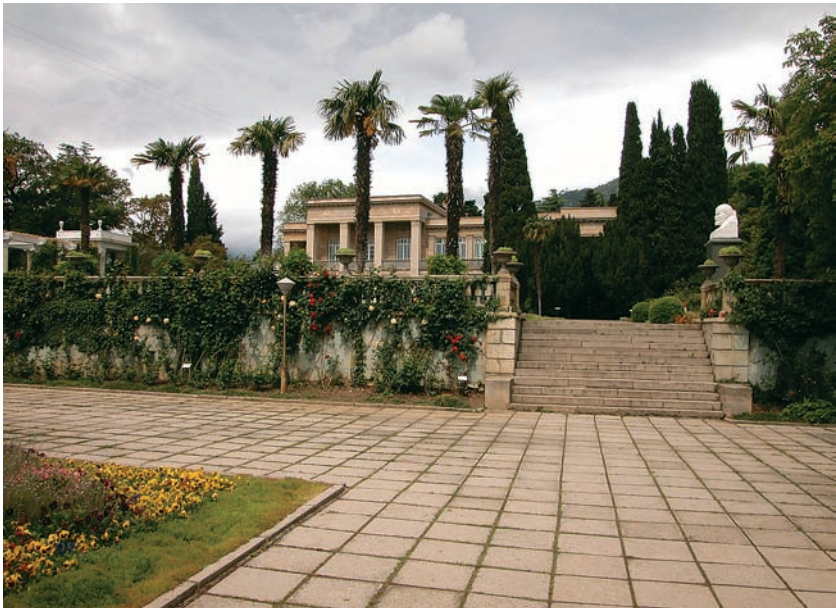
Fig. 84: Administration building of the Nikitsky Botanical Garden (site № 16, photo B. Prots)
