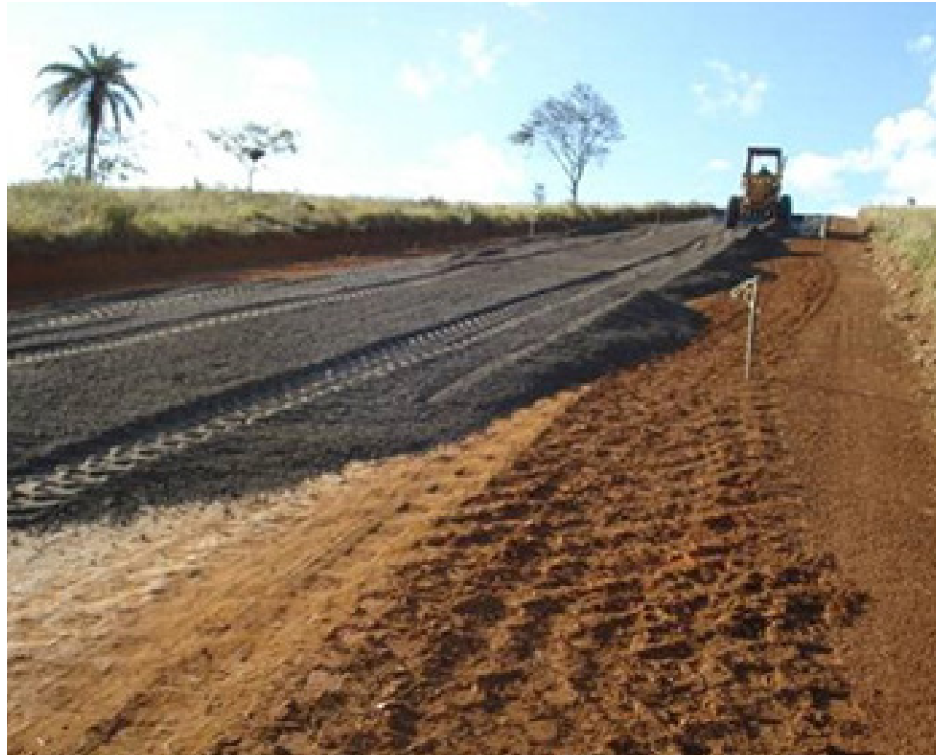
Road paved with Gerdau's co-products
