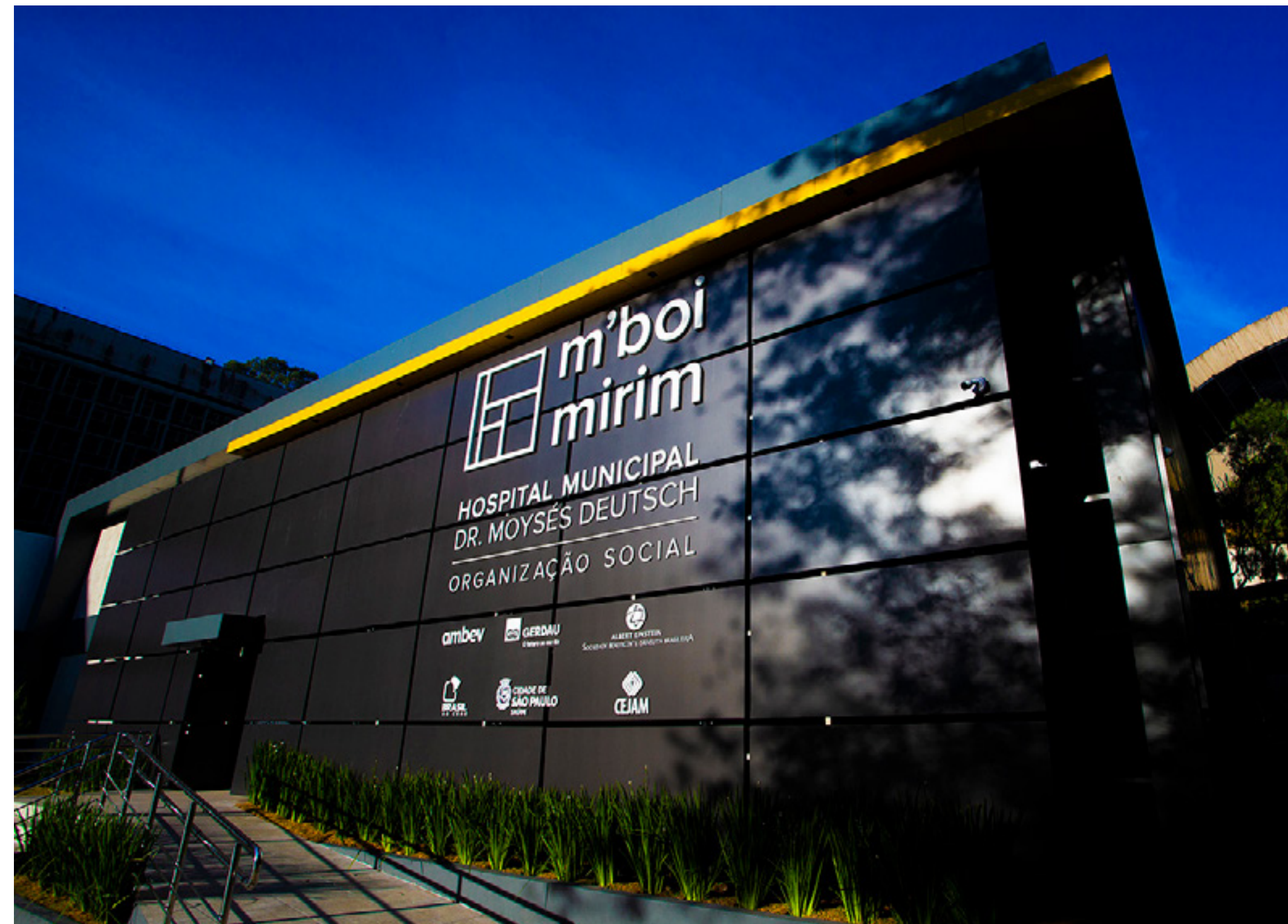
Covid-19 Treatment Center, in São Paulo (SP), built with resources from Gerdau and partner companies
