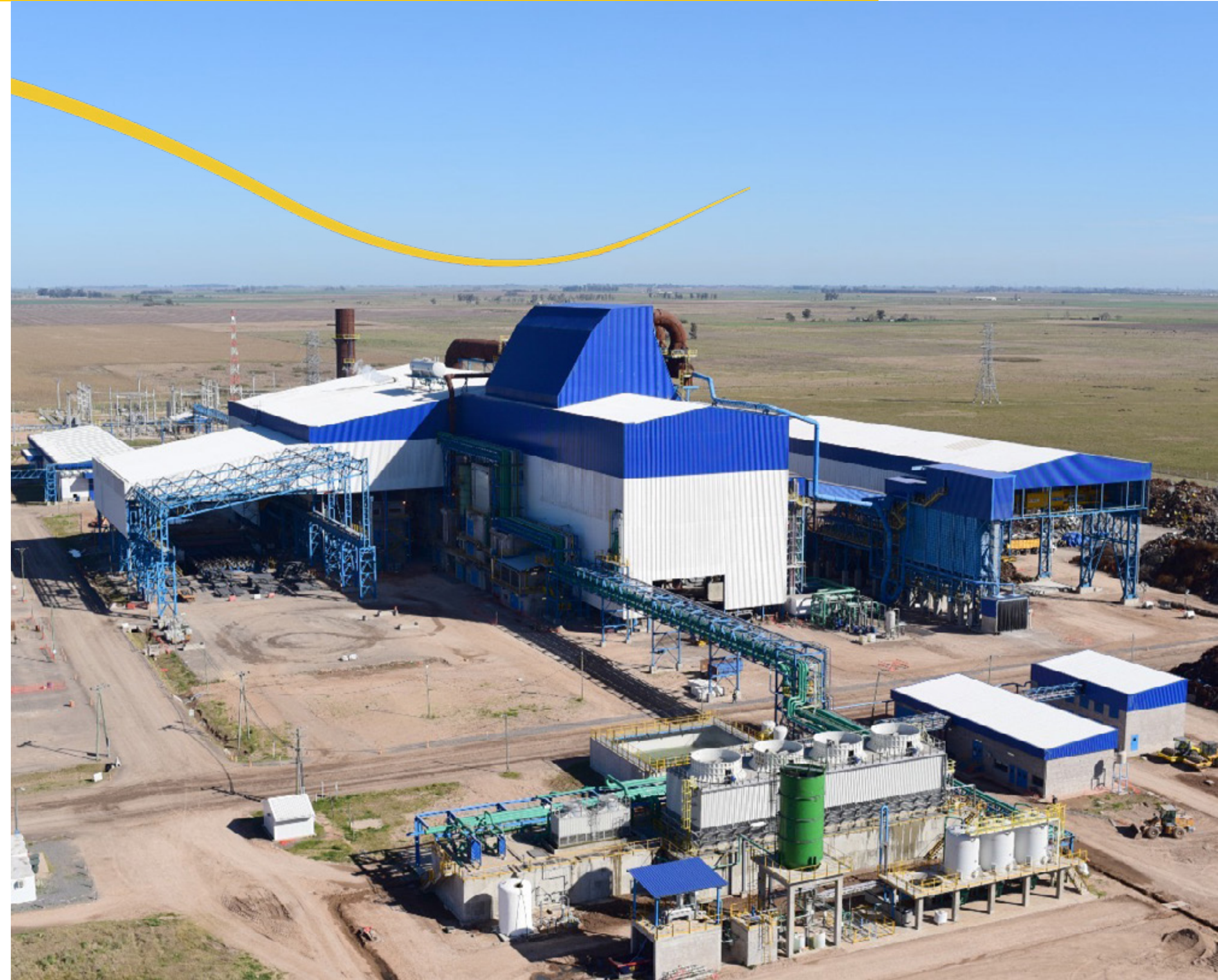
Gerdau's Melt Shop in Rosario, Argentina
