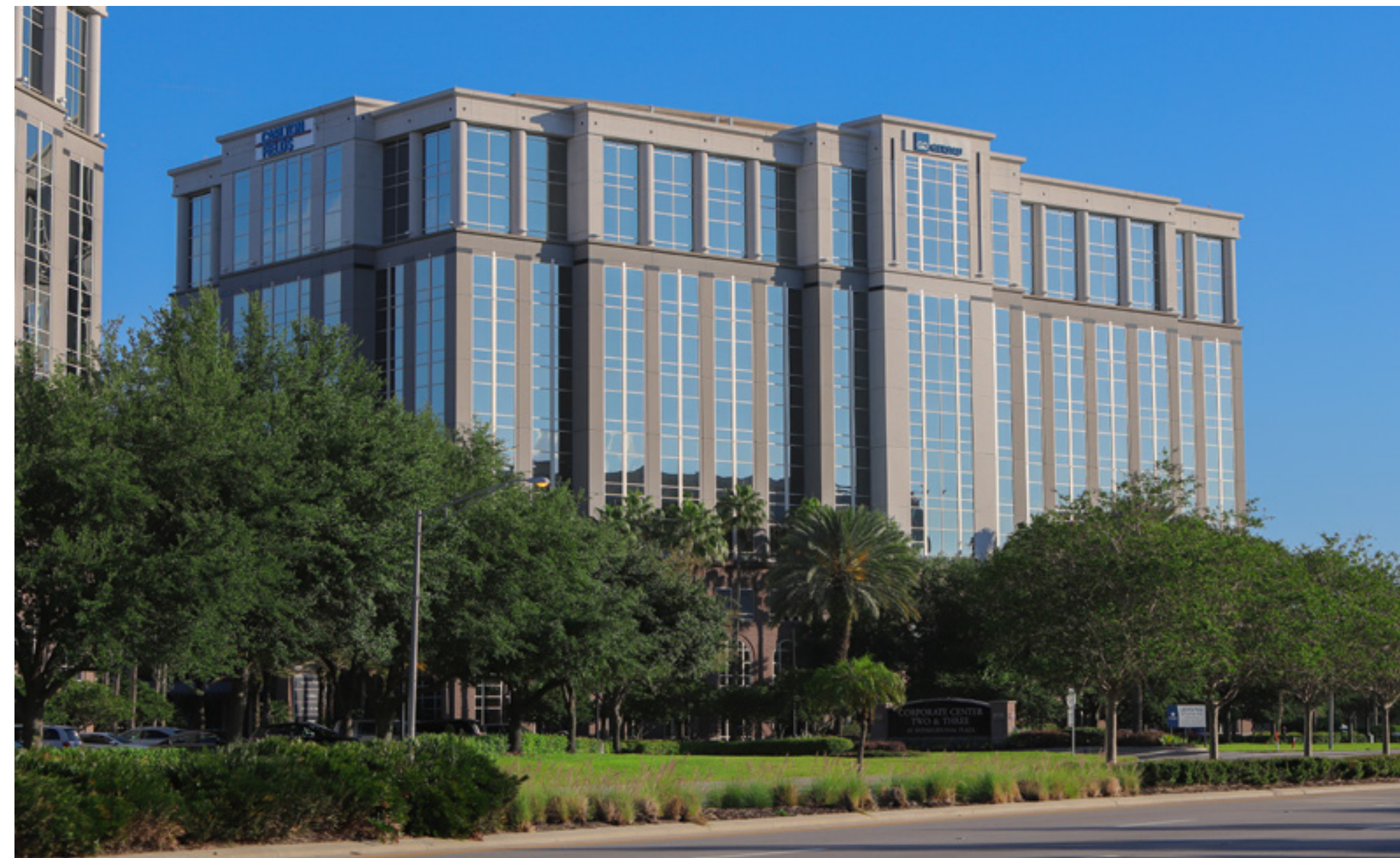
Gerdau office in Tampa, Florida (USA)
