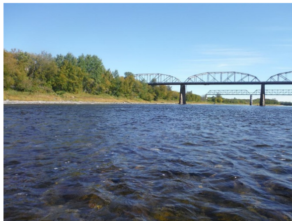
Photo 6 Fish Habitat within the Project Footprint Approximately 125 m Upstream of the Existing Bridge Crossing
