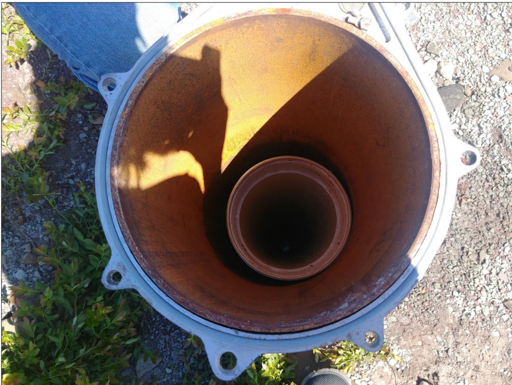
PHOTO 4 — View of insert in well 20-3. A similar insert is present in well 20-4.
