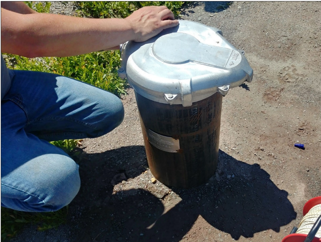
PHOTO 11 — View of well 20-4 (formerly Val-Doucet 3-1).
