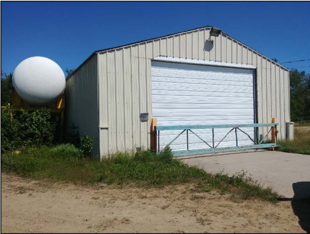
PHOTO 19 — View of building serviced by the Farm Well.
