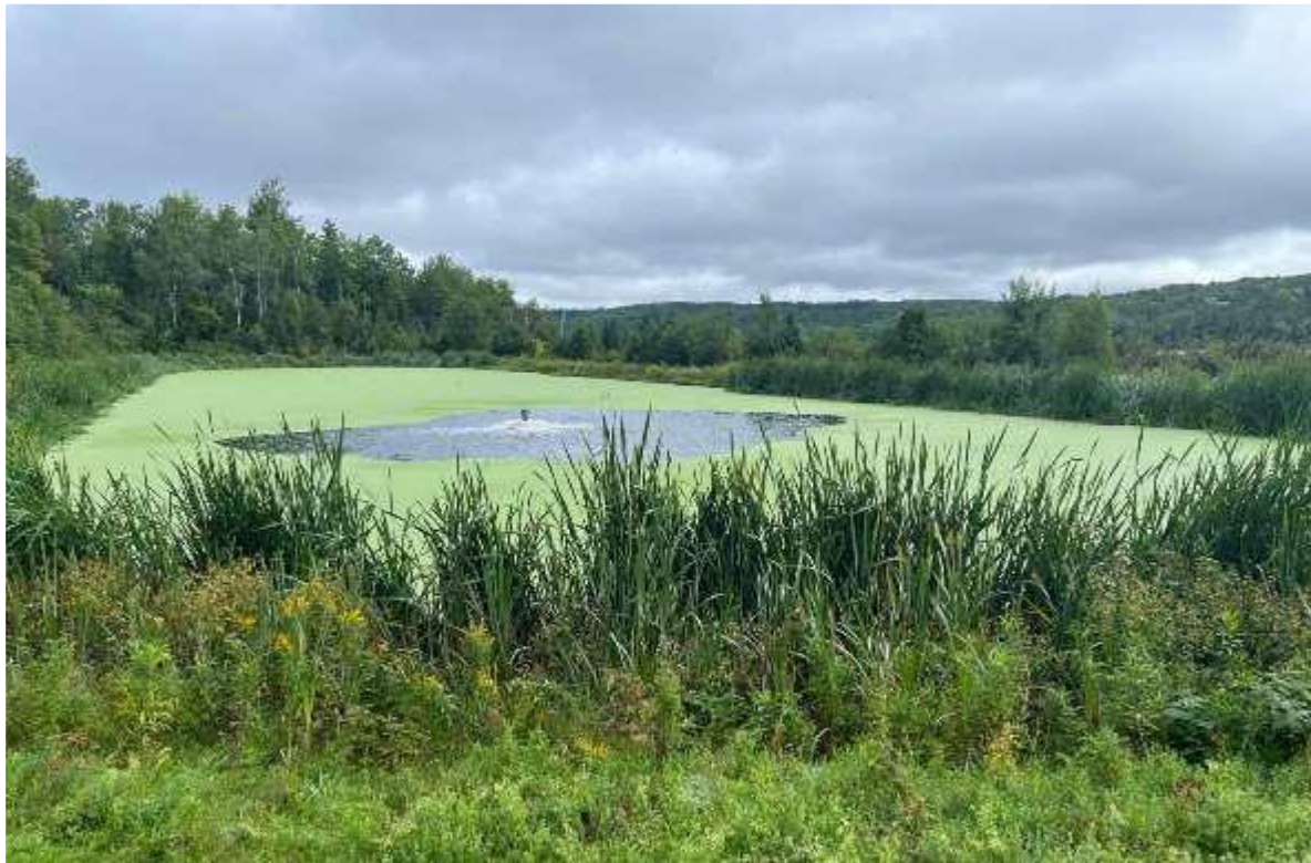
Photo No. 1: Existing Lagoon
