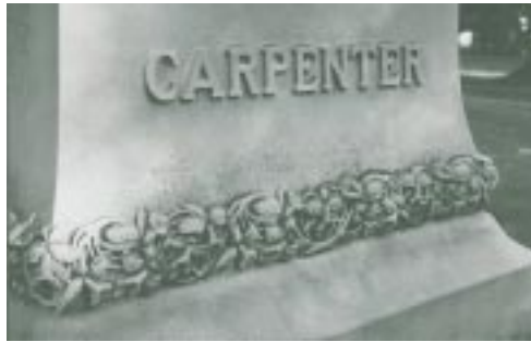
This complex floral frieze would cost upwards of $1000 per square foot to reproduce today.
