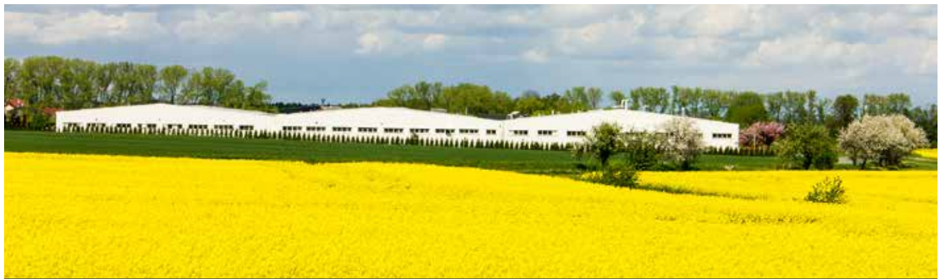
Year 2018 - a view from Dubany village to the new, already the fourth production hall for the ever-expanding production of wardrobes and special boxes
