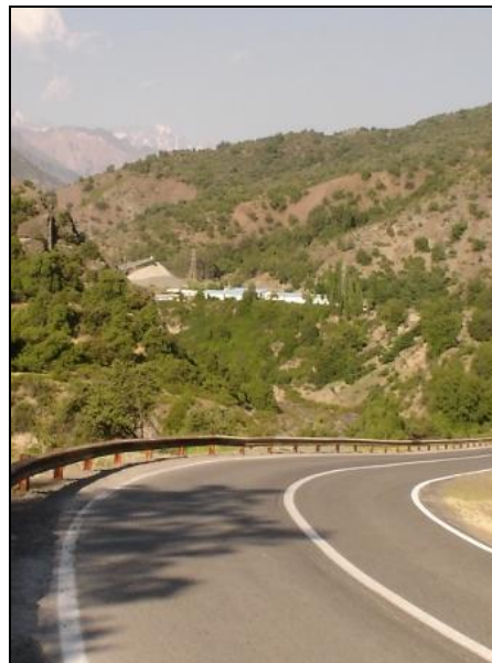
Picture 5.9.3.13 View towards NE in Colorado River valley in Río Colorado Mine.
