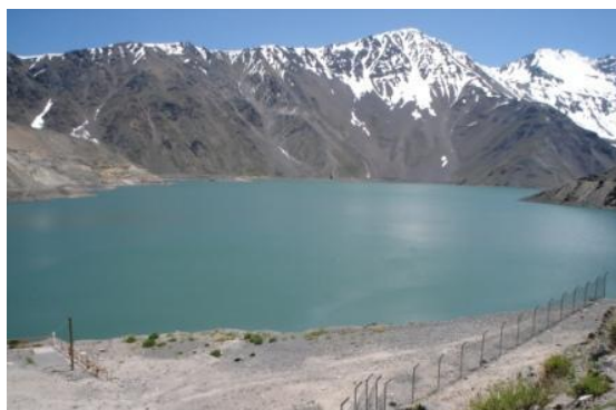
Picture 5.9.3.8 View towards N. El Yeso Reservoir close up
