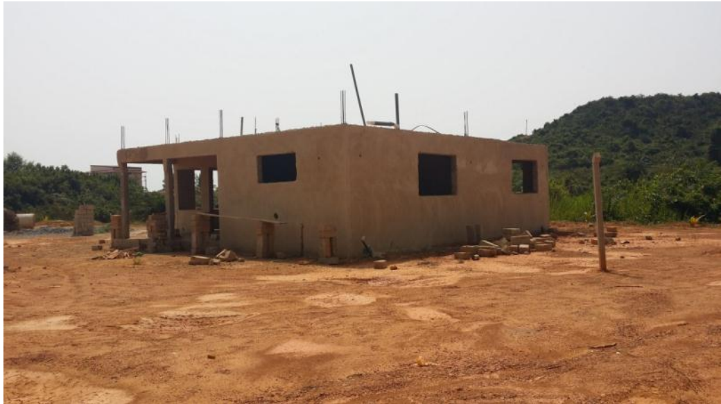
Figure 9.11: New Buildings West of Anankwari River – Single unit under construction
