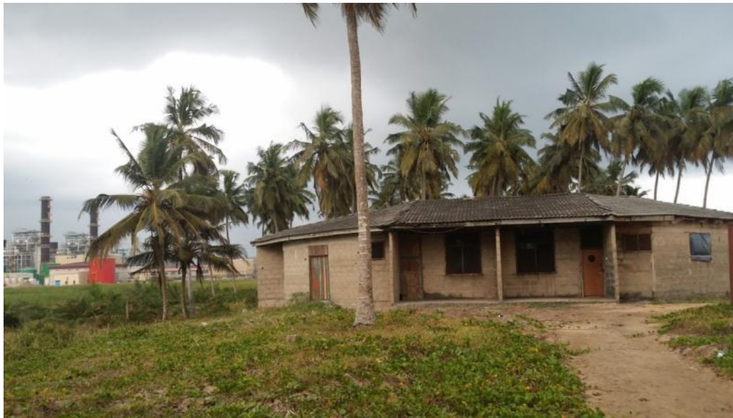
Figure 9.6: Structure to South-East of Project Site
