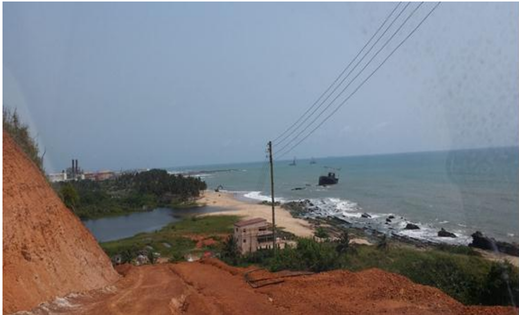
Figure 9.12: New Buildings West of Anankwari River – New beach house under construction (AEL’s Project site on the far side)
