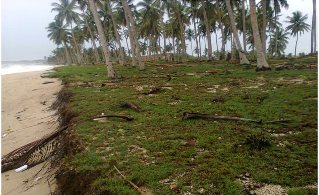
Figure 10.2 – Coastal Erosion at Aboadze
