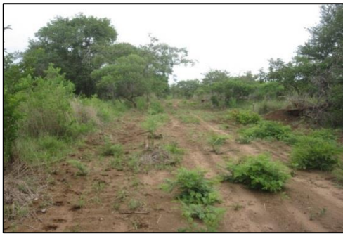
Figure 17: Cleared powerline corridor through woodland
