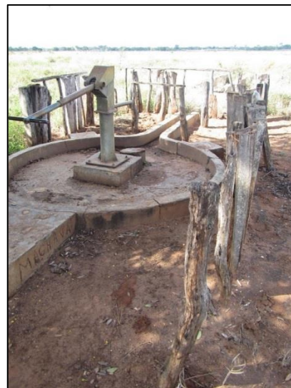
Figure 52: Hand pumps have been installed close to some villages to provide drinking water tom local people
