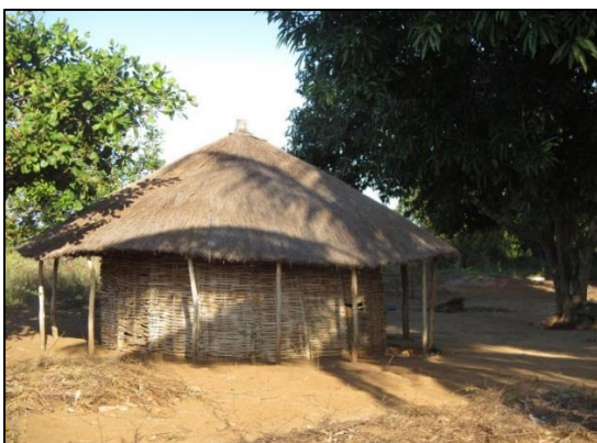
Figure 38: Hut built out of local sourced natural material including, thatching grass, wood and reeds
