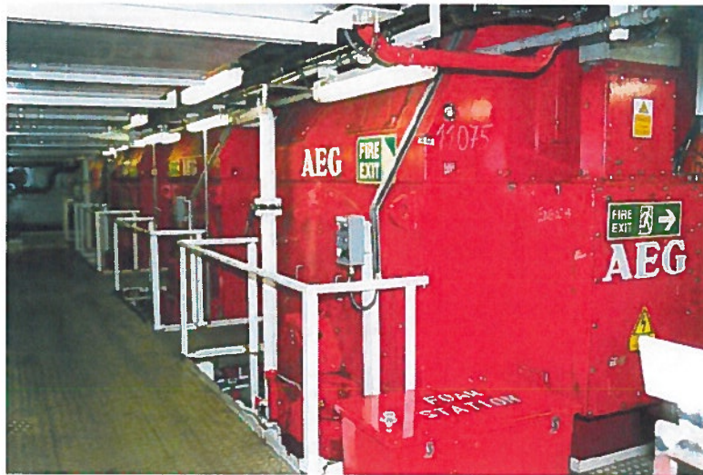
Diesel generators 1-4
