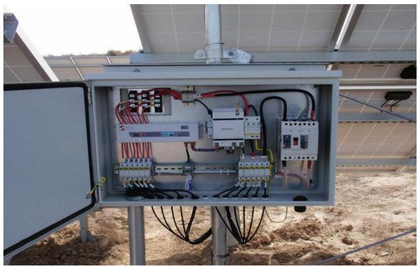
Figure 3.8: Combiner Box Attached to the Mounting Structure of a Solar Panel.
