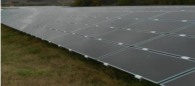
Plate 2.4: Typical Appearance of Thin-Film CdTe Arrays Source: OST Energy (First Solar)
