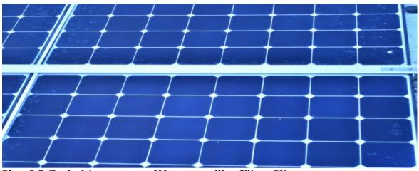
**Plate 2.5: Typical Appearance of Monocrystalline Silicon PV arrays** Source: OST Energy
