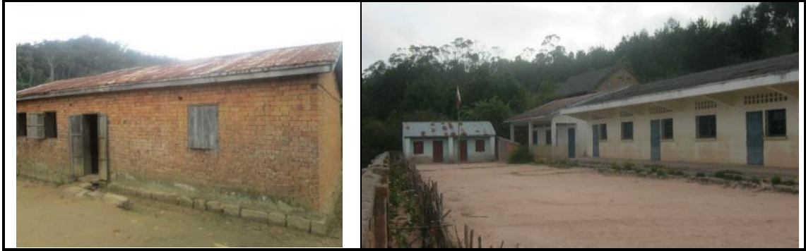
Photo 13 - Antenina Primary School and Tsinjoarivo Secondary School
