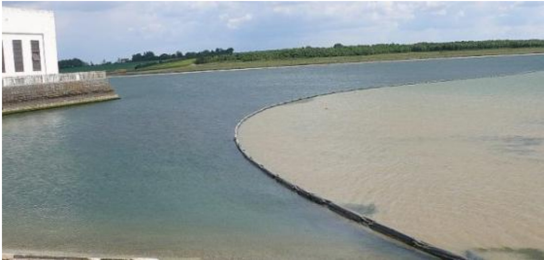
Photograph II.3. 65. Silt curtains that prevent turbidity
