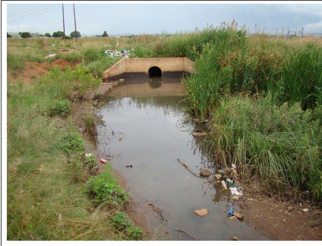
Photograph3. An artificially created seasonal pond has been created for stormwater attenuation. Ideally the seasonal pond should be rehabilitated and used for stormwater attenuation for the proposed commercial and residential developments.
