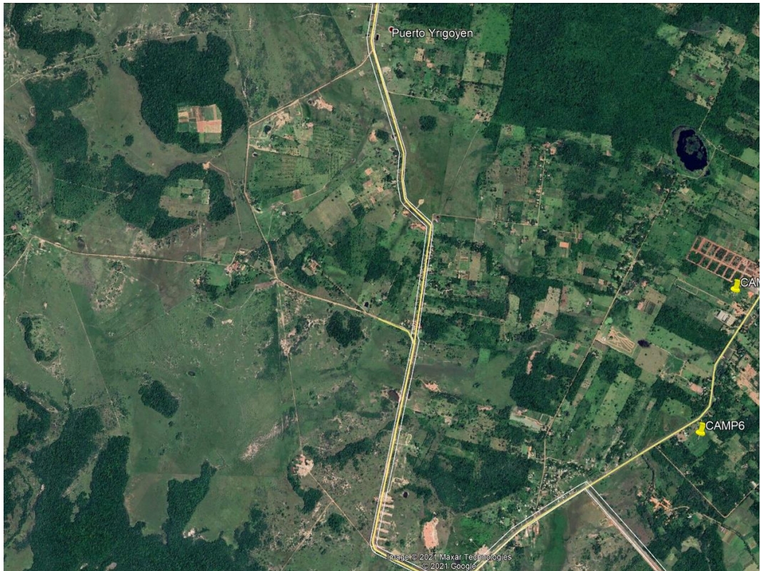
Figure 11 – Transmission Line Sections 3/5 (from the mill). Image: Google Earth jul/2021.
