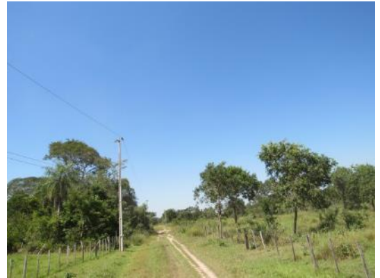
Figure 130 – Another unpaved access angle present in DIA. Coordinates UTM - 21k 449021.77 E/7430667.35 S (P1).
