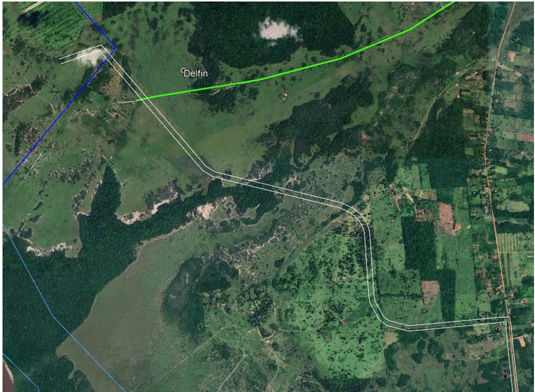
Figure 9 – Transmission Line Sections 1/5 (from the mill). Image: Google Earth jul/2021.
