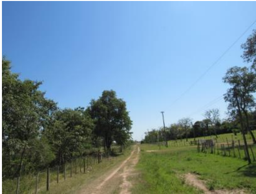
Figure 129 – View of the unpaved access present in the DIA. Coordinates UTM - 21k 449021.77 E/7430667.35 S (P1).
