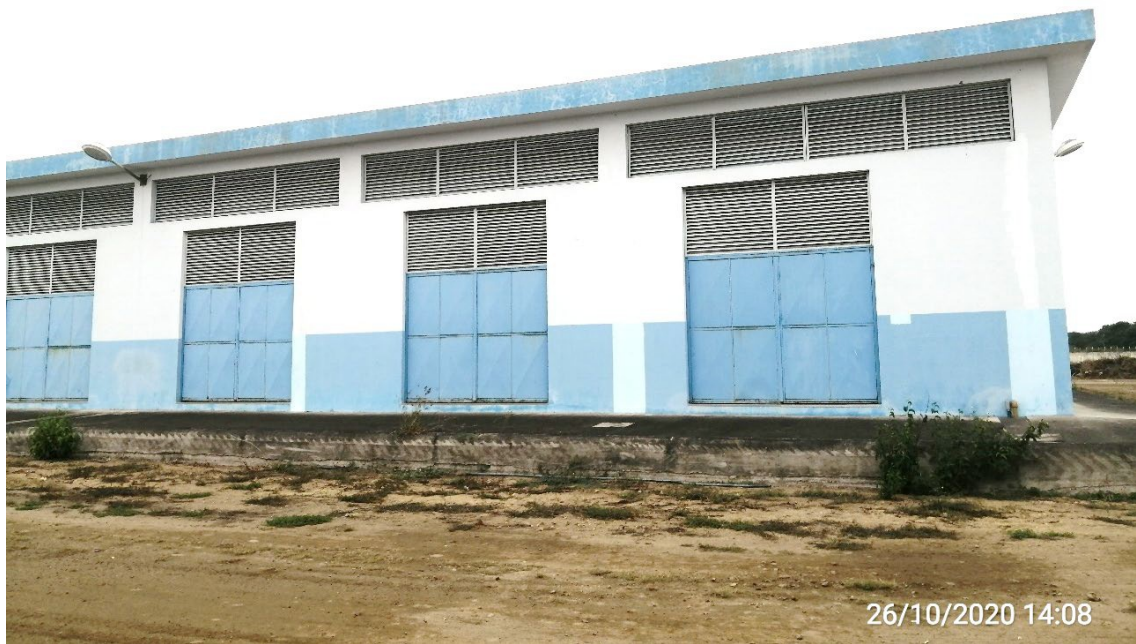
Emergency generator room, built in 2012
