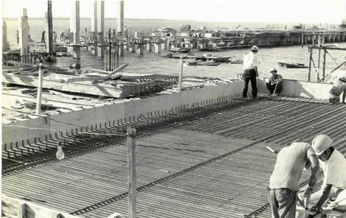
Construction of the breakwater pier, year 1962
