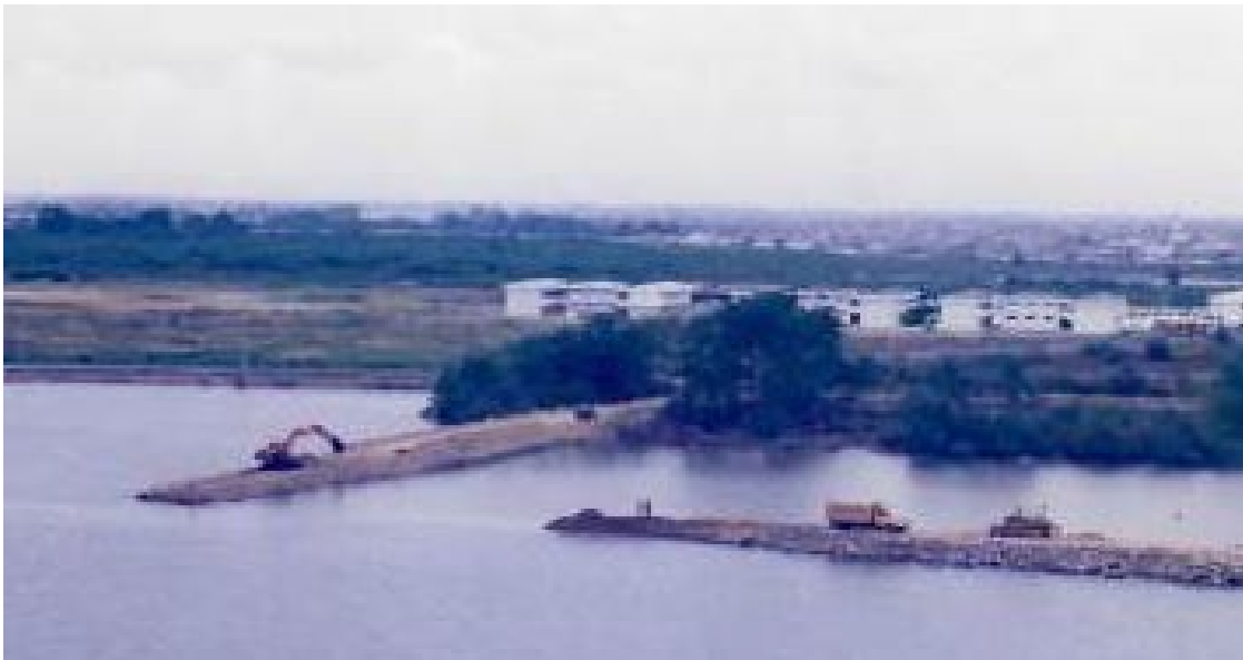
Work for the consolidation of the current Yard area No. 10, year 2012.
