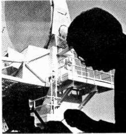
*A Bell Labs scientist silhouetted against Bell's new millimetre-wave aerial. This sensitive radio antenna is being used, according to Bell, to study "the highest frequency signals ever continuously beamed down to earth from orbiting satellites." The experiments will help tell if these higher frequency signals, from two satellites transmitting at 19 and 28GHz, could be used reliably for future satellite systems. A third satellite will join them in May next year.*
