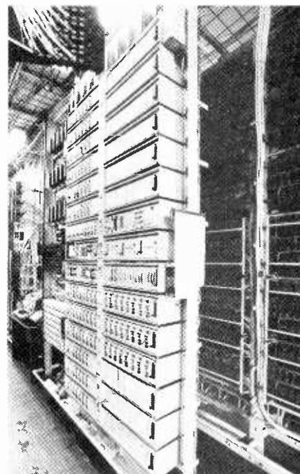
The prototype electronic director at Surbiton. This equipment rack replaces 14 of the electromechanical type. The equipment has a translation store of 2,000 individual routing instructions, any of which can be rewritten using a keypad, providing for the routing of traffic to several hundred local exchanges, to the trunk network or various information centres. The translators are installed in triplicate in case of failure, but there have been no faults on the equipment in two years.
