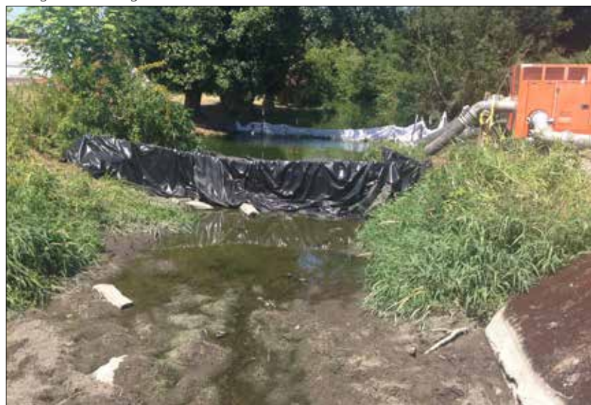
Figure 28. This channel was dewatered to replace a downstream culvert. Water was pumped around the project area to allow for access. Mussels were salvaged and relocated before the area was dewatered, during the fish salvage, and during the final drawdown.
