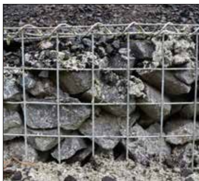
Figure 25. Gabion baskets are commonly used to protect infrastructure on slopes and banks but can limit habitat and vegetation.
