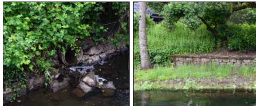
Figure 24. Left: Retaining walls that cover banks and are built up from the streambed limit mussel habitat. Right: When walls are set back from the water's edge, a larger area of natural shoreline is retained, which can provide better mussel habitat.
