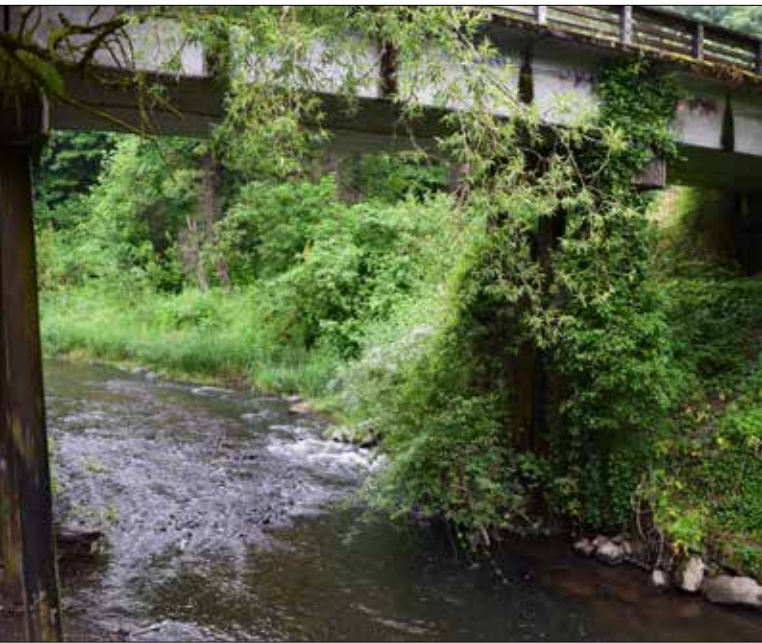
Figure 19. Bridge footings that span streams reduce the need for riprap, as seen along the right bank, that makes for poor mussel habitat unless sediment readily accumulates.
