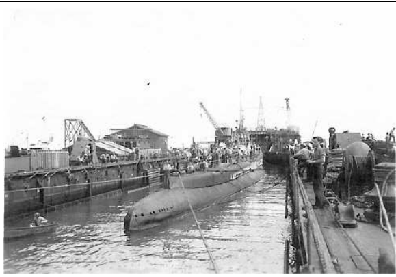
ARD-8 floating drydock, flooded to allow a submarine in the dock, date unknown, Midway Island
