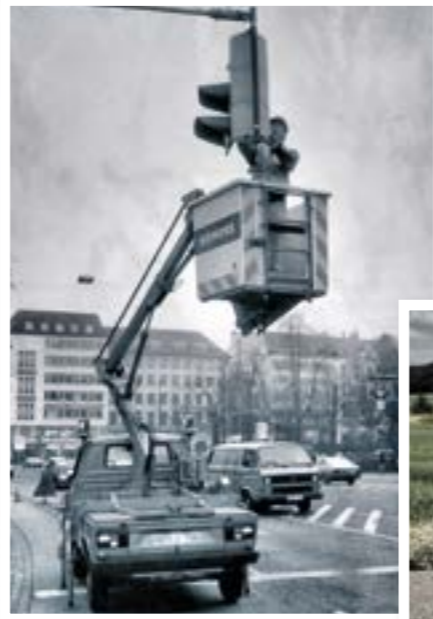
This cherry-picker is perfect for changing bulbs in overhead traffic lights.
