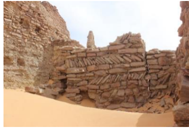
Figure 12. The wheat spike method in Agham N'khzin Ksar Aghlad (photos by Y. Kassou).
