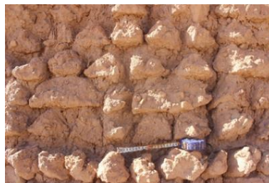
Figure 13. Triangular prism mud walls in Agham Tidji Ksar Kali (photos by Y. Kassou).
