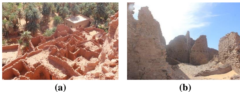
Figure 11. Rubble stone on fortified walls: (a) Built walls with Tafza in Agham Tihdayine Ksar Faroun; (b) Built walls with slate stones in Agham At-Youcef Ksar Aghlad (photos by Y. Kassou).
