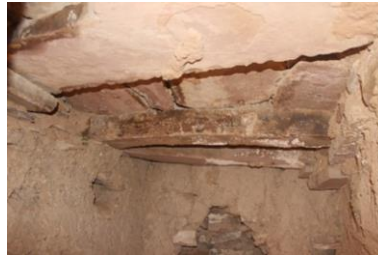
Figure 19. Roofing with stones in Ksar Aghlad (photos by Y. Kassou).
