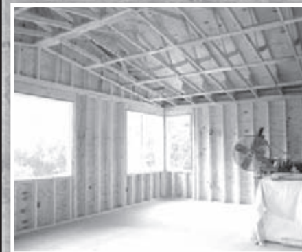
Home addition, during
