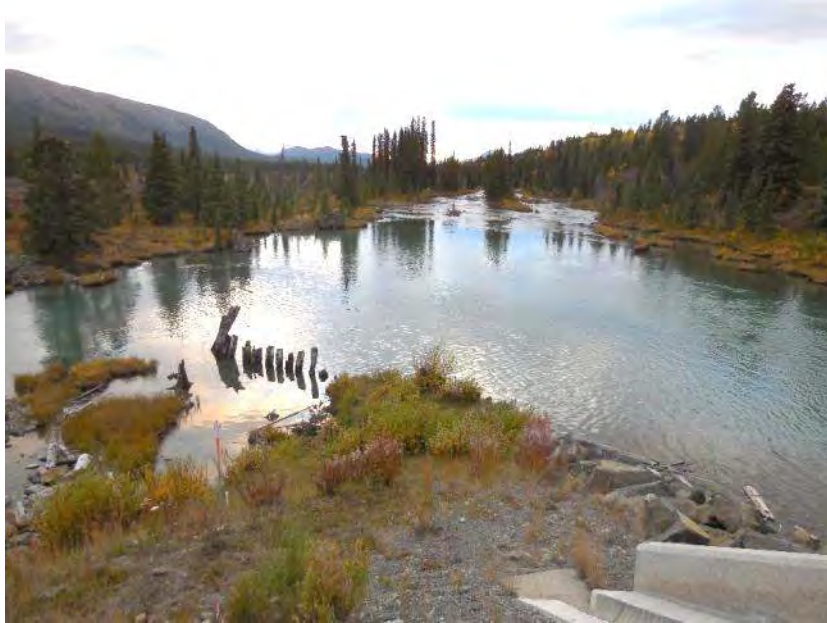
Photo 11: Pine Creek looking downstream from Surprise Lake control structure
