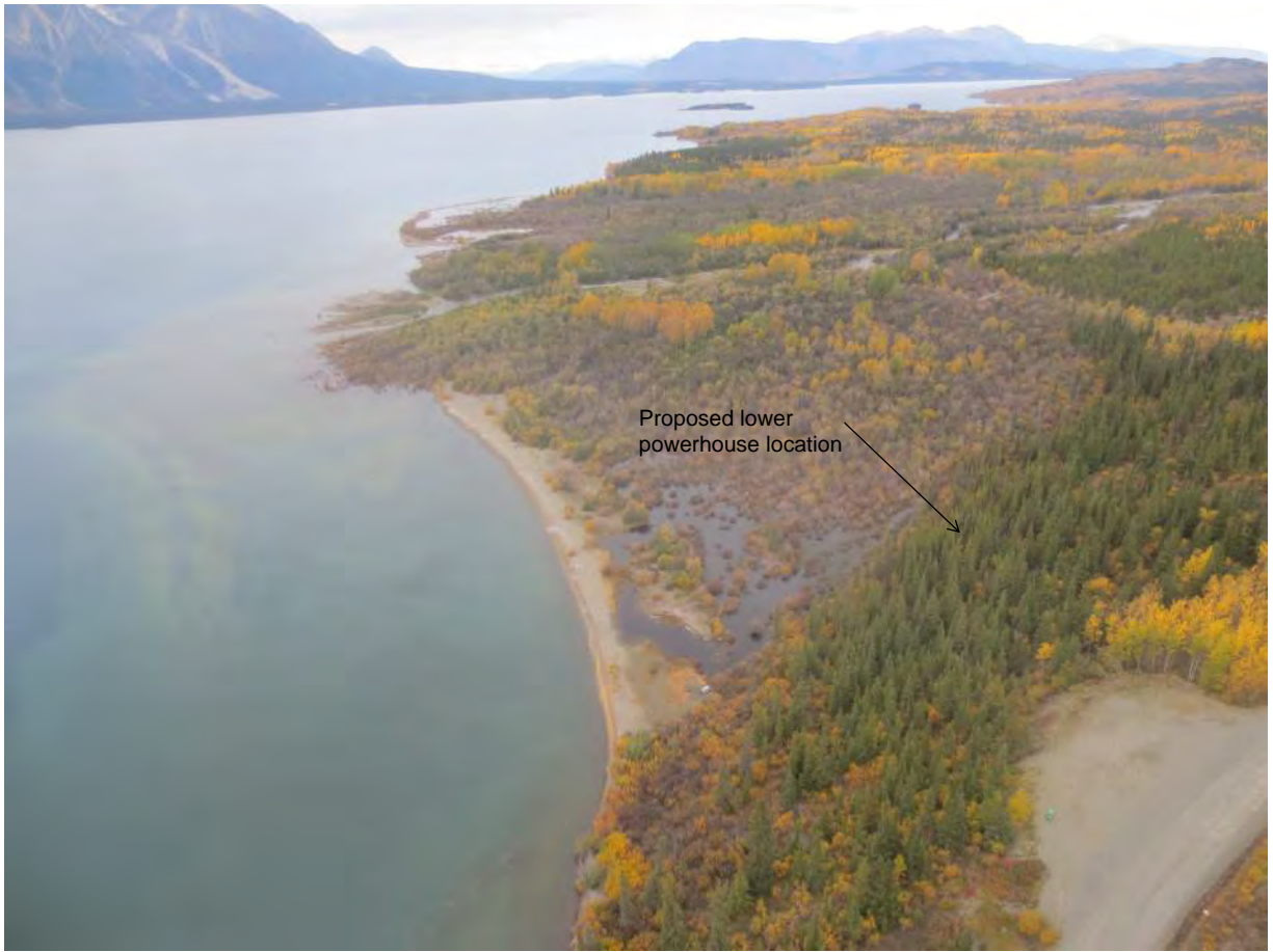
Photo 5: Proposed lower powerhouse location, looking north.
