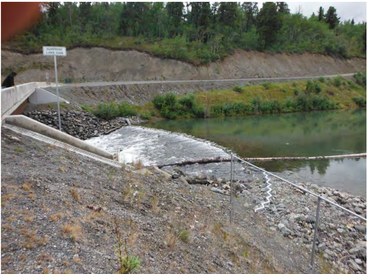
Photo 2: Surprise Lake rockfill weir, looking north.
