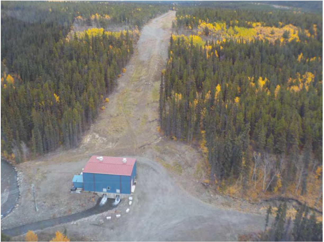
Photo 3: Existing powerhouse looking east towards penstock right of way
