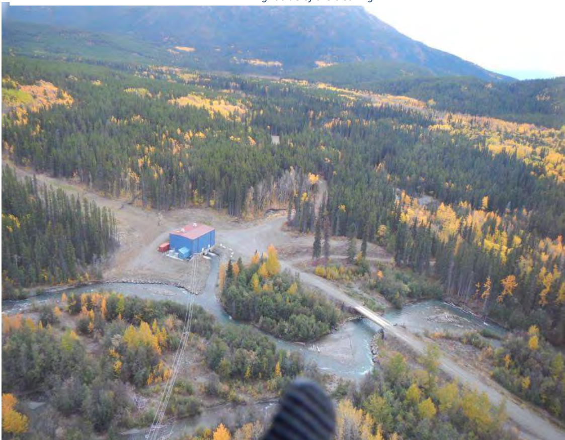
Photo 3. Existing powerhouse looking south towards Spruce Creek. Pine Creek is in foreground.
