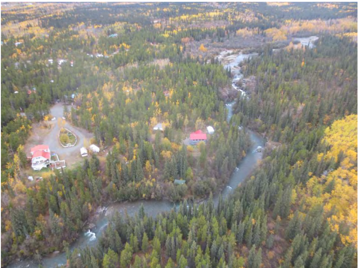
Photo 6: Lower cascade on Pine Creek, looking upstream. Proposed lower penstock alignment would be on right side of photo.
