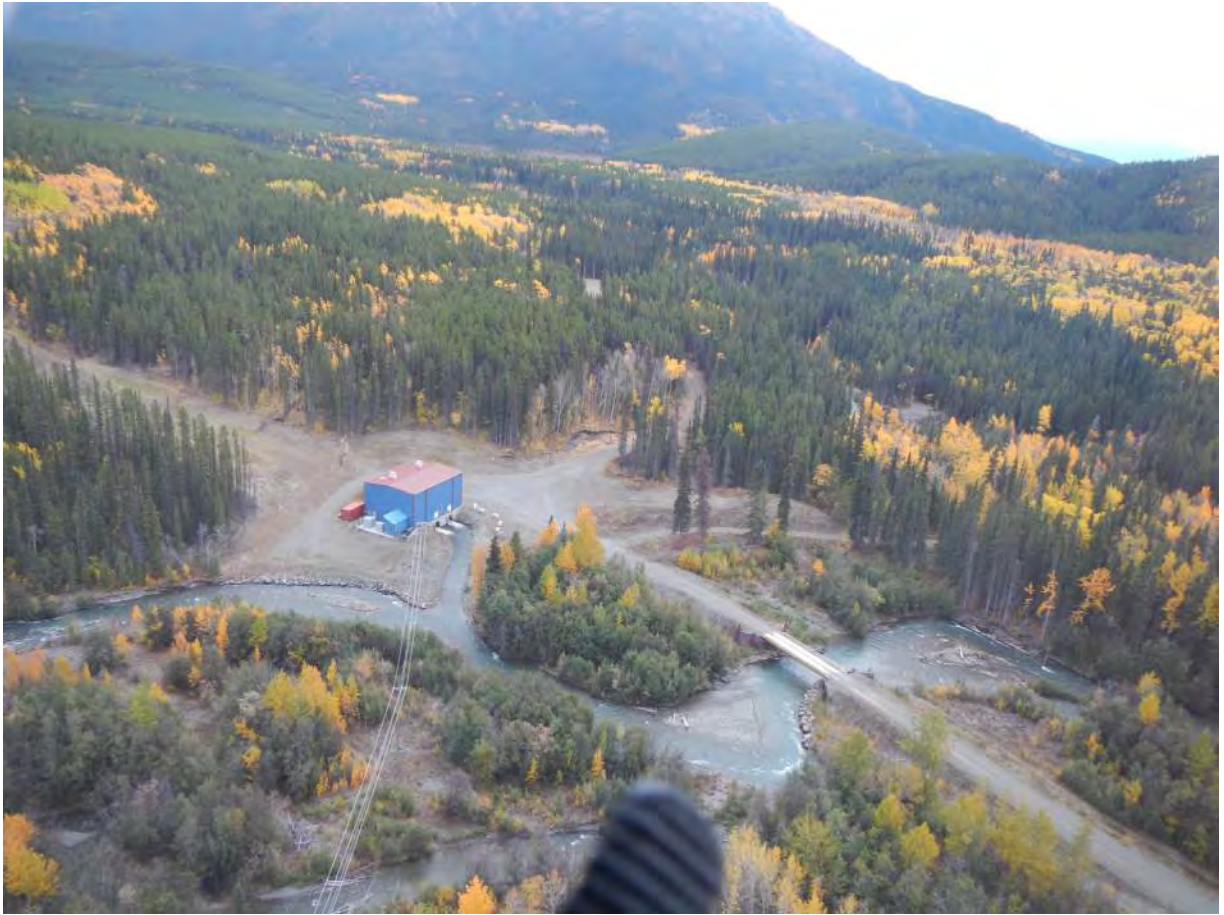
Photo 5: Overview of existing powerhouse area and access road.
