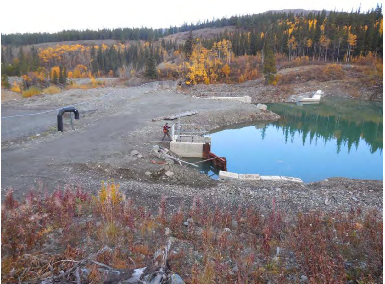
Photo 4: Existing intake structure.
