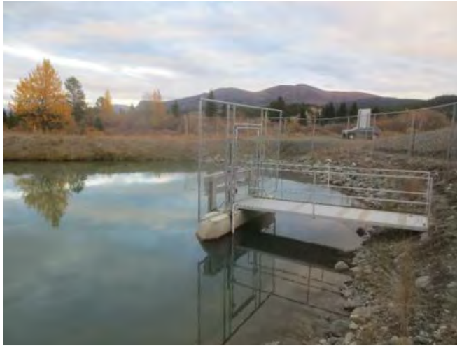
Photo 8: Existing outlet structure at Surprise Lake
