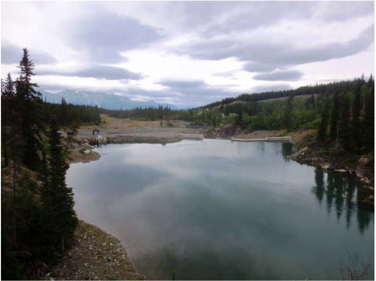
Photo 3: Existing head pond, weir and existing intake structure, looking west.
