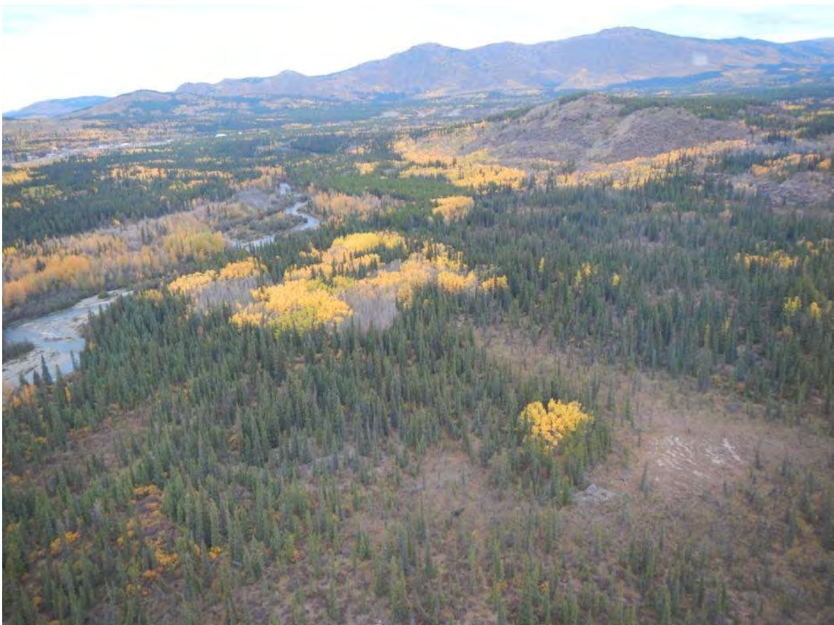
Photo 5. View of lower penstock alignment terrain conditions looking north towards existing powerhouse.
