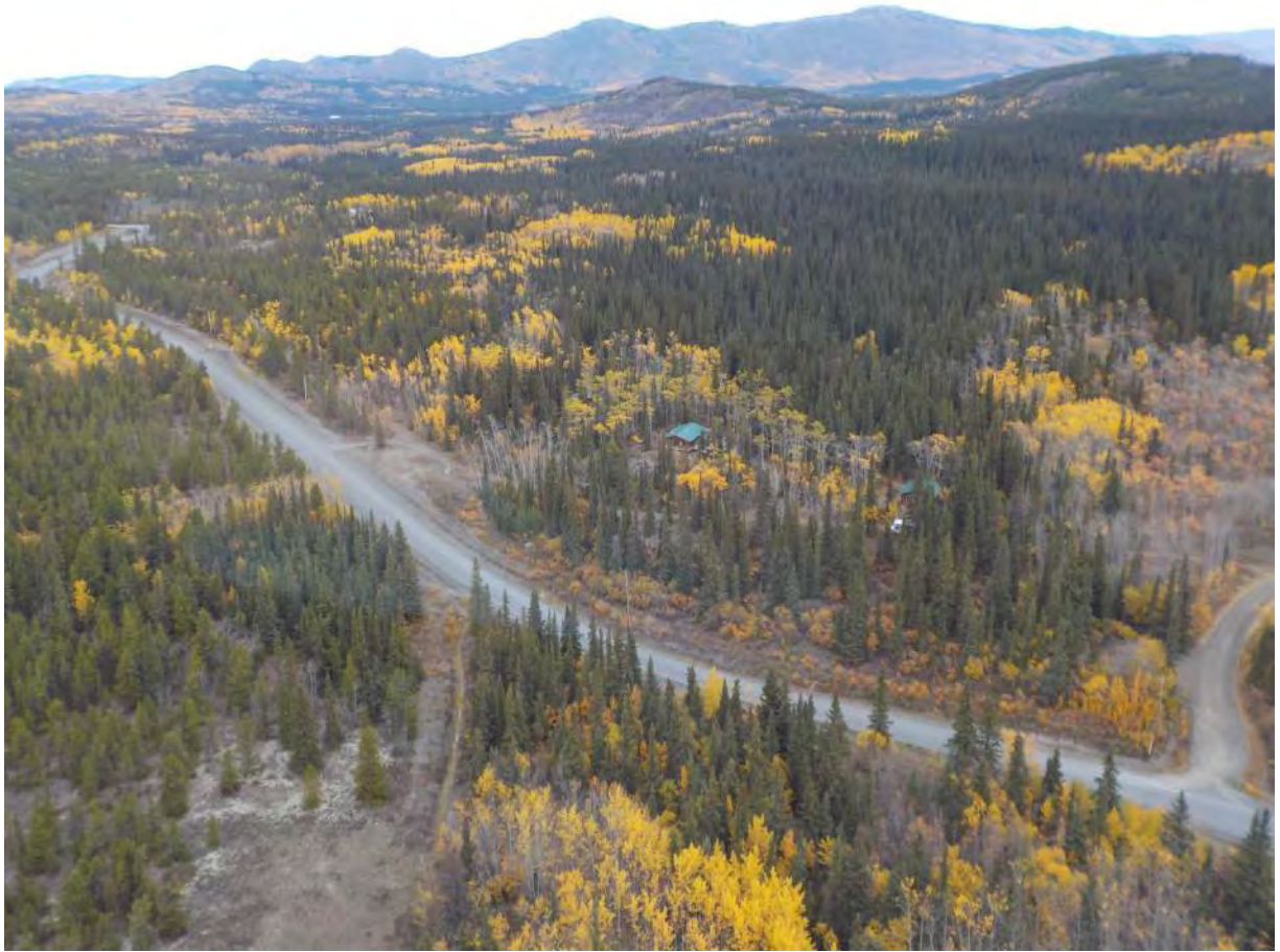
Photo 7: Bottom portion of lower penstock alignment, looking east. Warm Bay Road in foreground with Arts Centre Road on the right.
