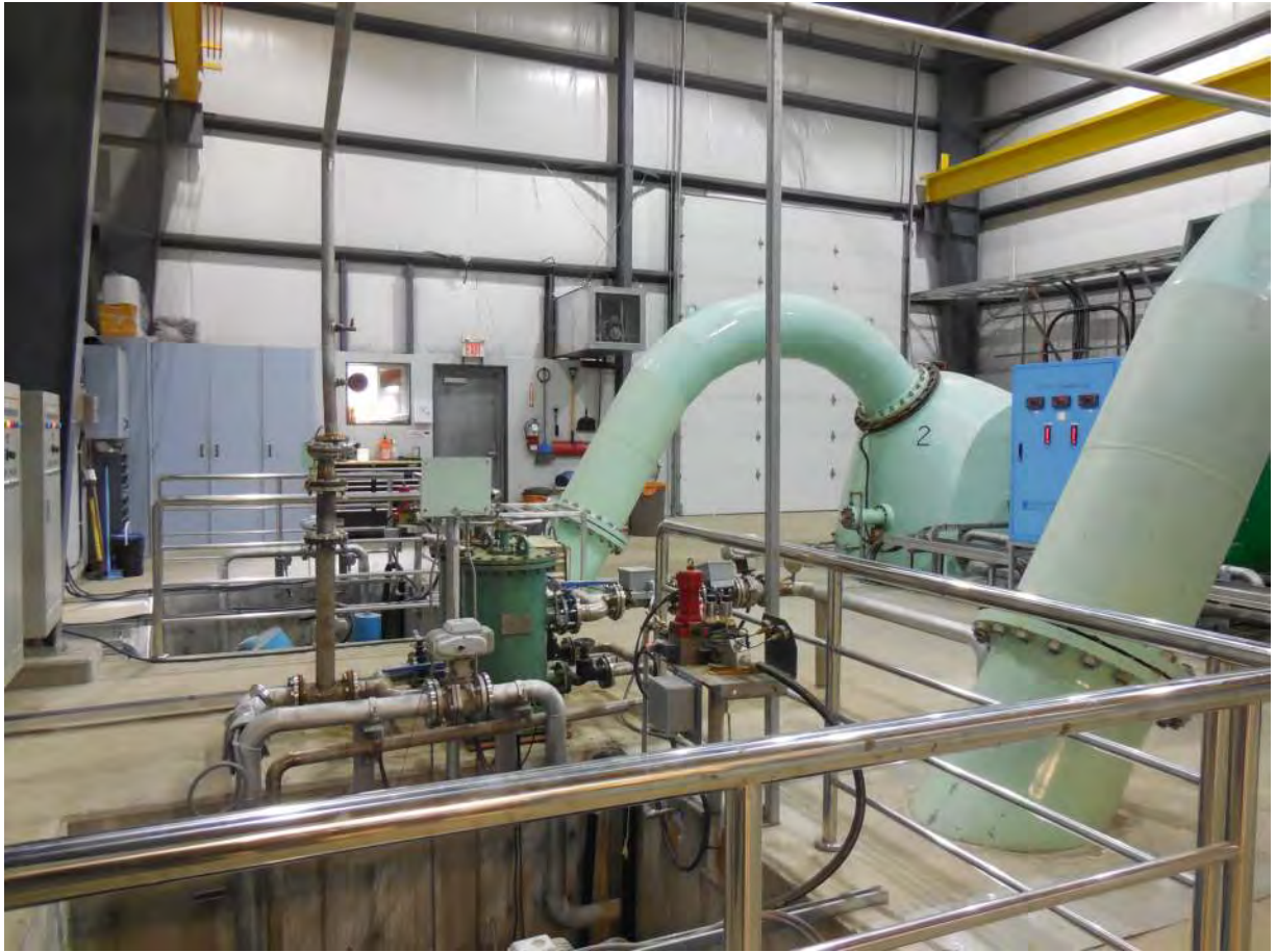
Photo 9: Interior view of south wall of powerhouse.
