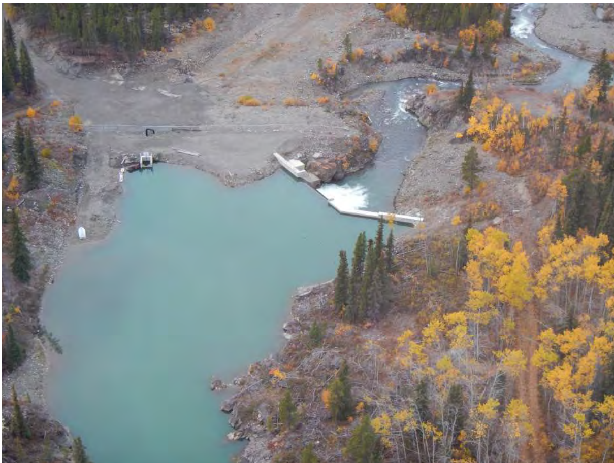
Photo 2: Existing head pond, weir and existing intake structure, looking downstream.
