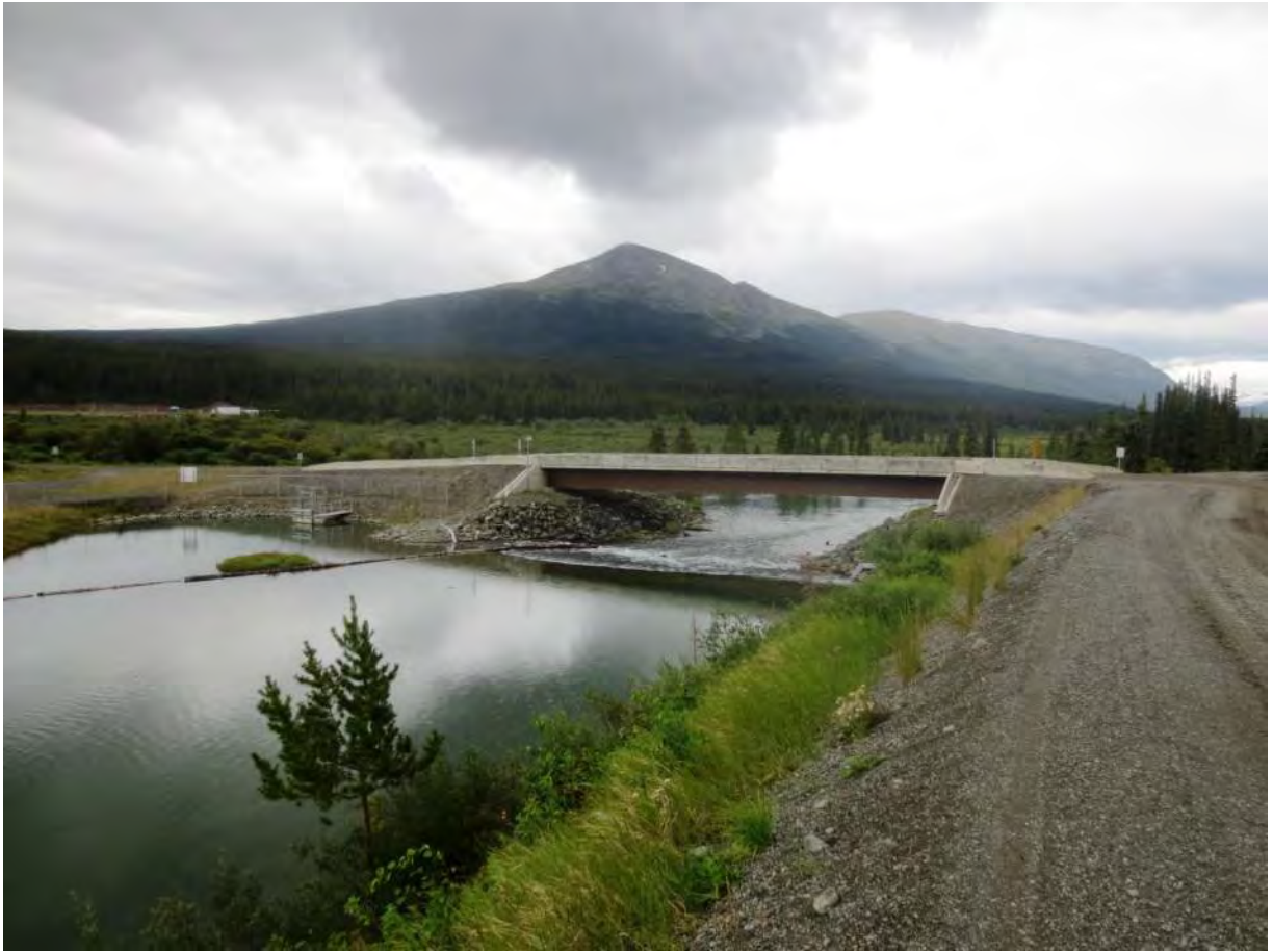
Photo 1: Existing rockfill weir looking downstream. Outlet structure on the left.
