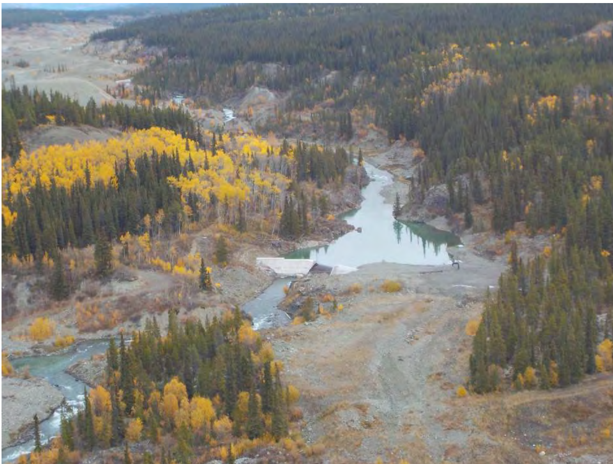
Photo 1: Existing (upper) head pond, looking upstream. Note placer mine workings upstream.
