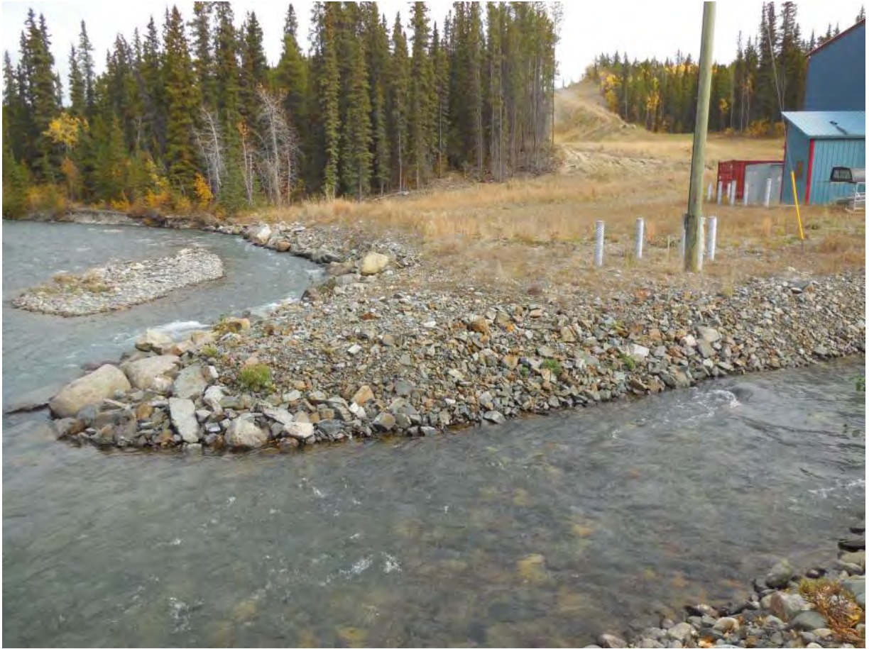
Photo 7: Tailrace confluence with Pine Creek, looking east. Existing powerhouse is to right of photo
