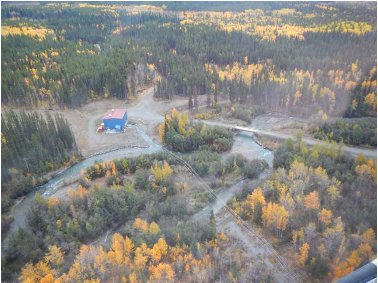
Photo 1: Proposed lower head pond location downstream of existing access road bridge
