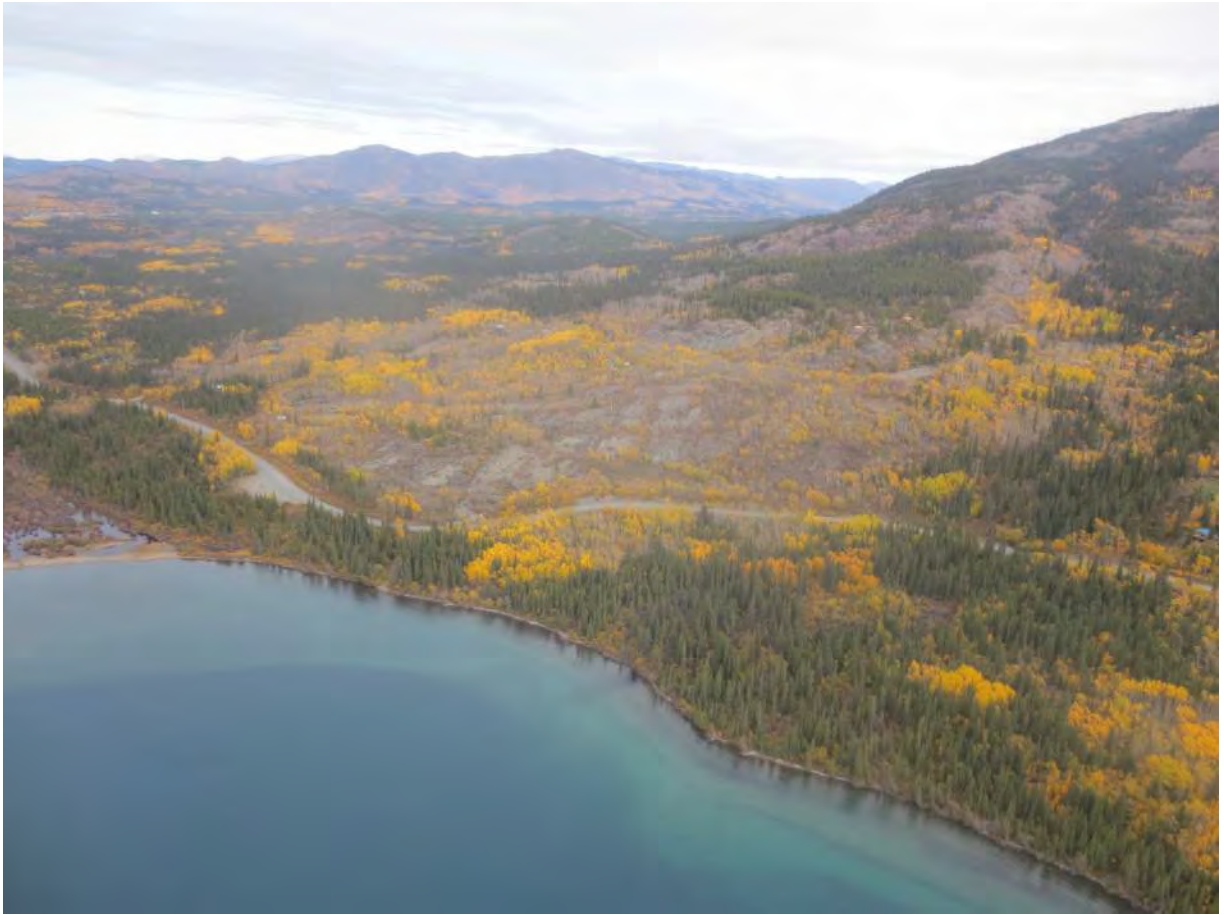
Photo 3: Proposed lower powerhouse location, looking northeast. Alternate location considered is on the right hand side of photo.
