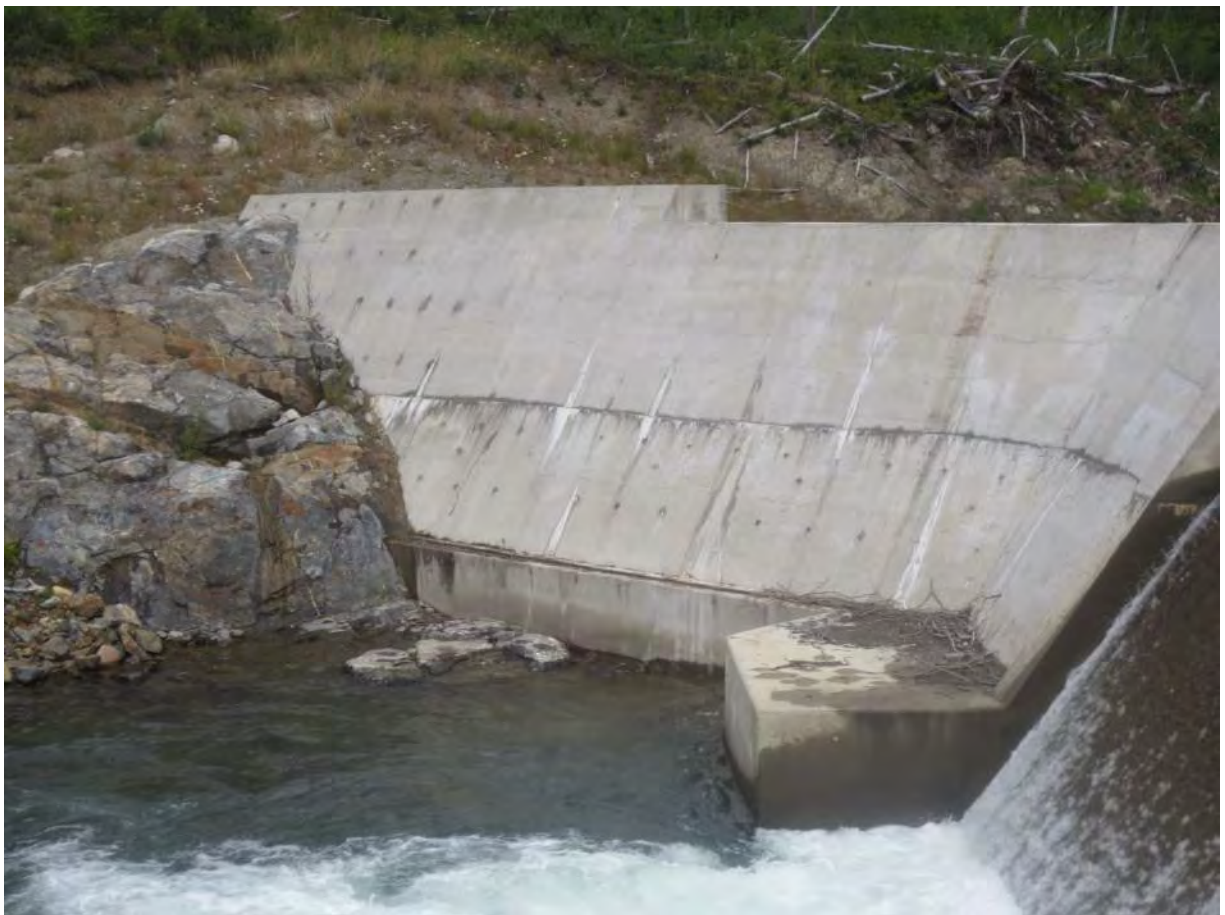
Photo 8: North abutment of weir.
