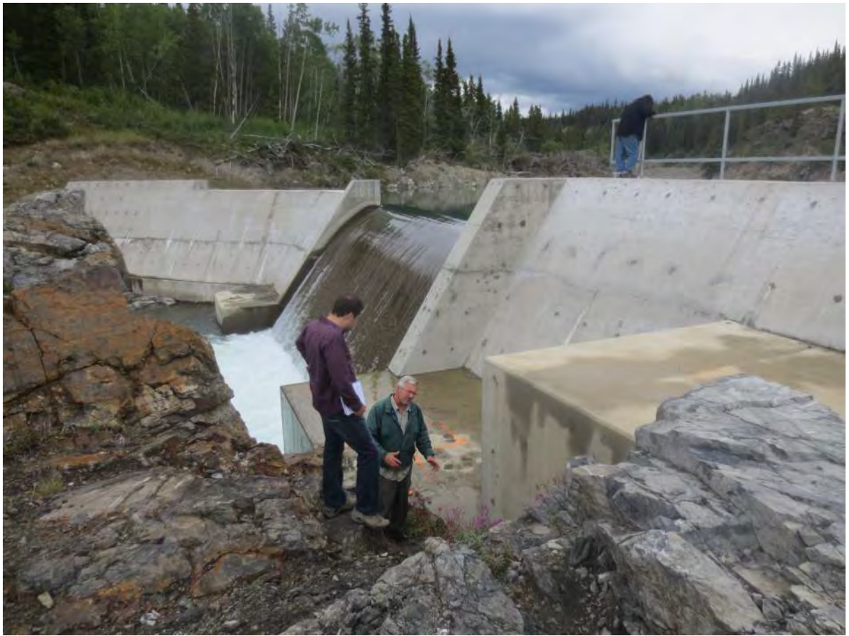
Photo 7: Downstream side of weir.
