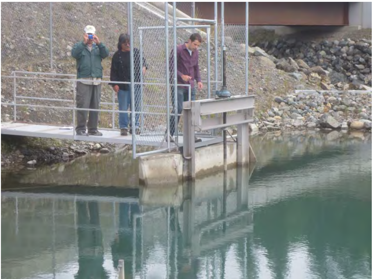
Photo 4: Existing outlet structure at Surprise Lake.
