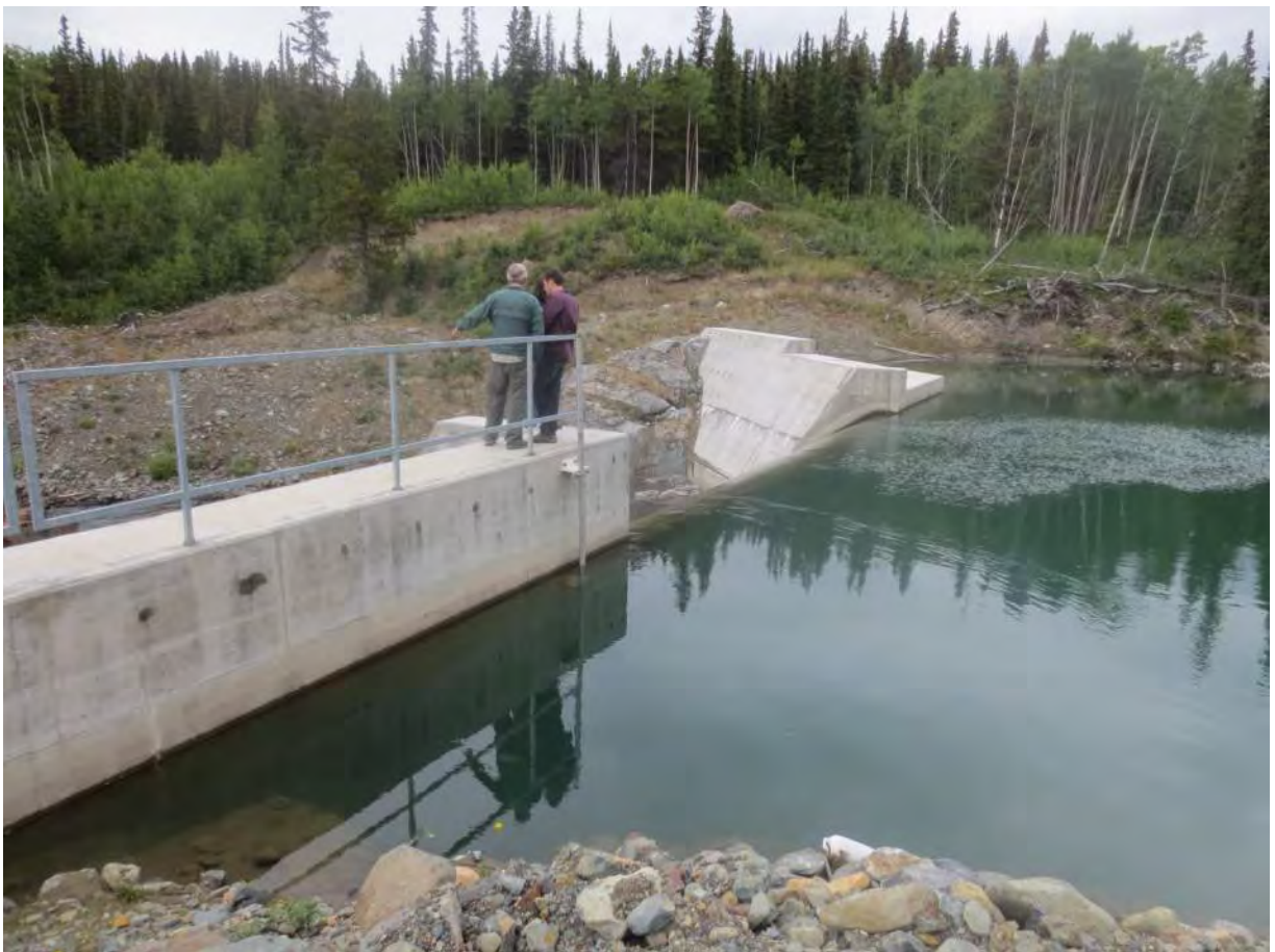
Photo 6: Upstream side of weir.
