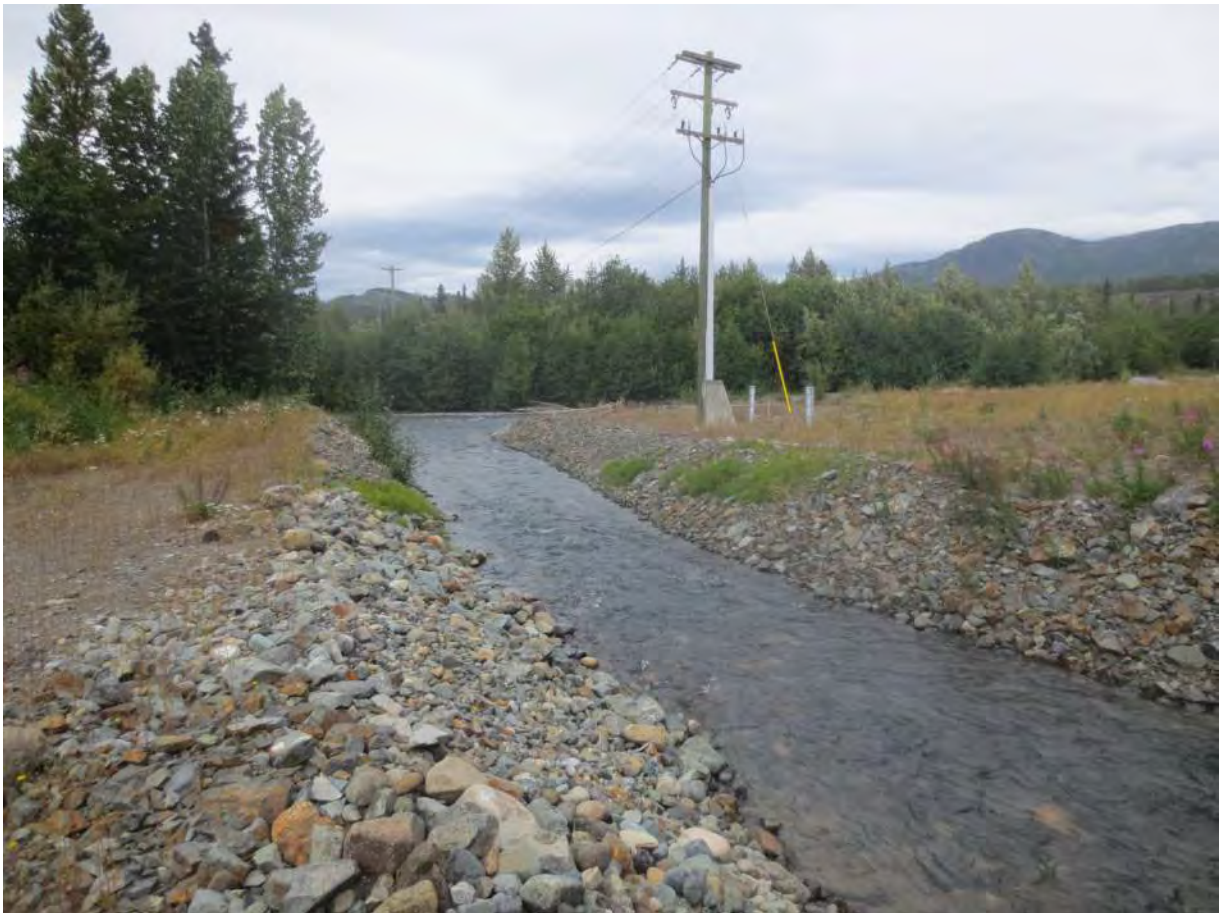
Photo 6: Tailrace exiting powerhouse towards Pine Creek
