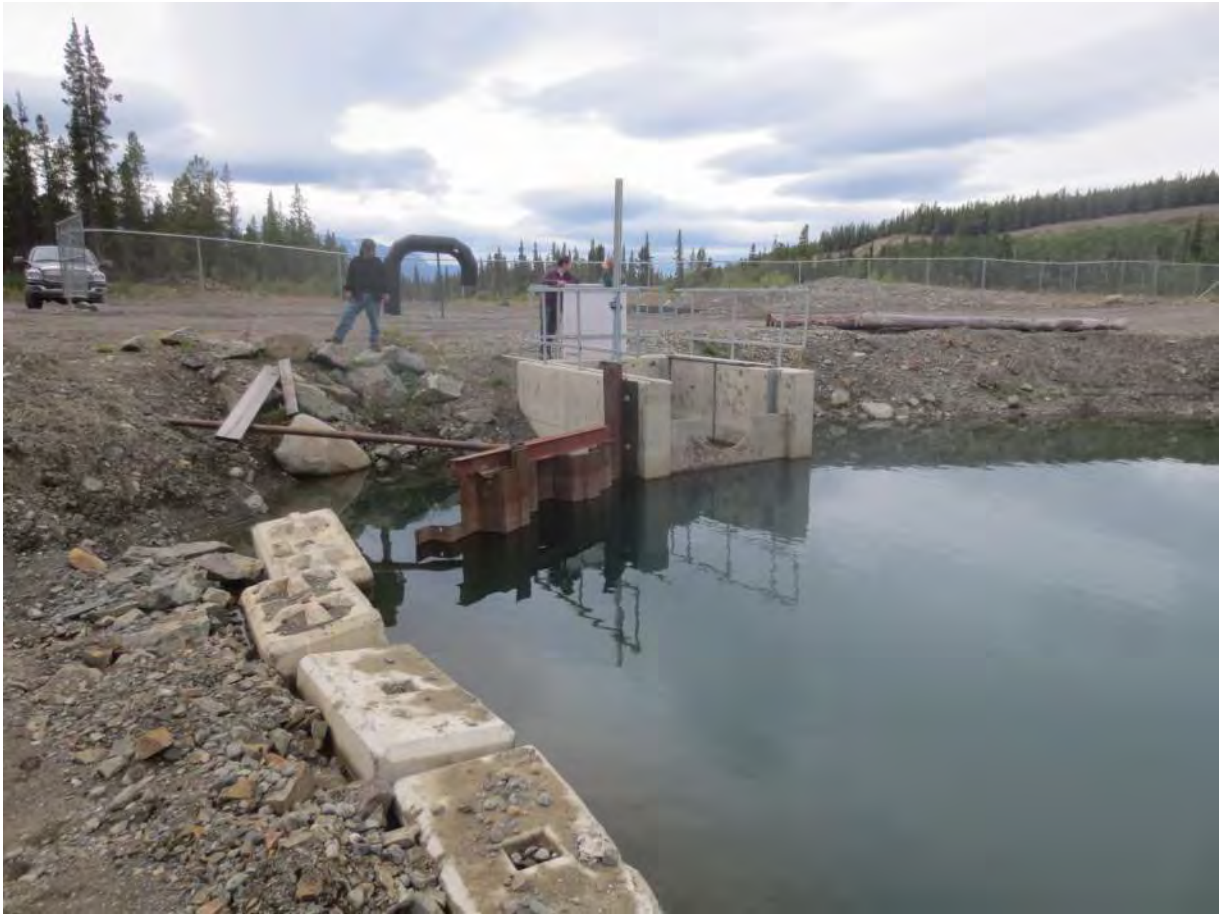
Photo 5: Existing intake structure.
