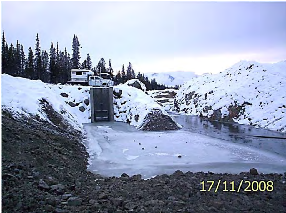
Photo 12: Existing intake under construction with diversion channel to the right
