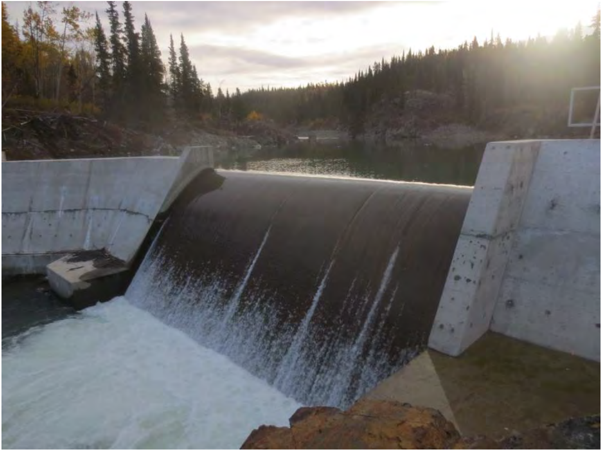
Photo 9: Overflow section of weir.
