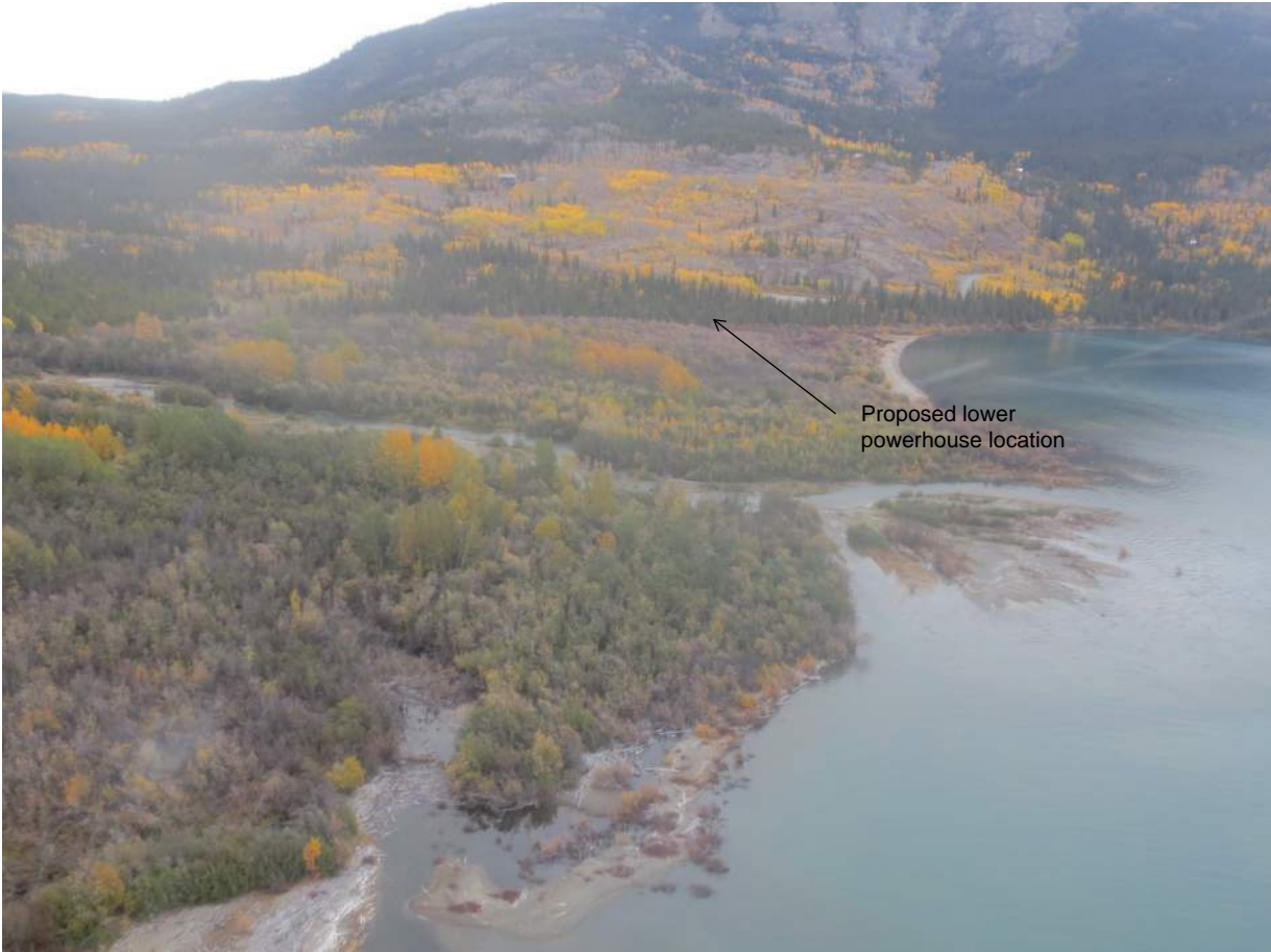
Photo 2: Mouth of Pine Creek looking south towards proposed lower powerhouse location.
