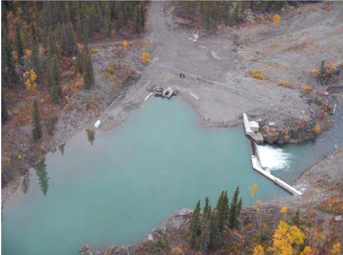
Photo 2: Existing head pond and intake structure, looking west.
