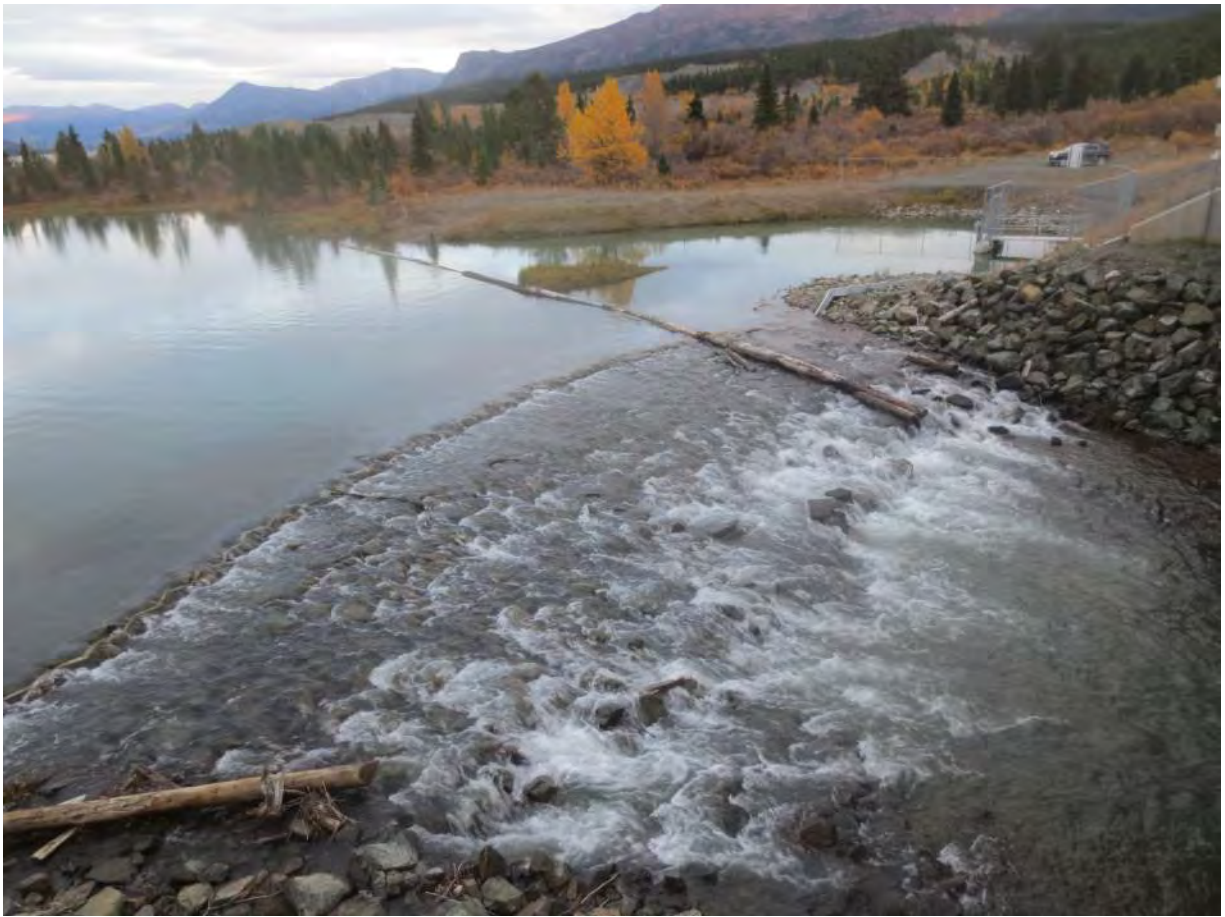
Photo 3: Surprise Lake rockfill weir, looking south towards outlet structure
