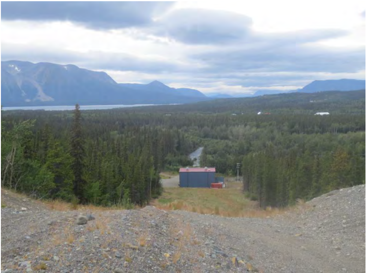
Photo 4: Existing powerhouse looking west from penstock right of way
