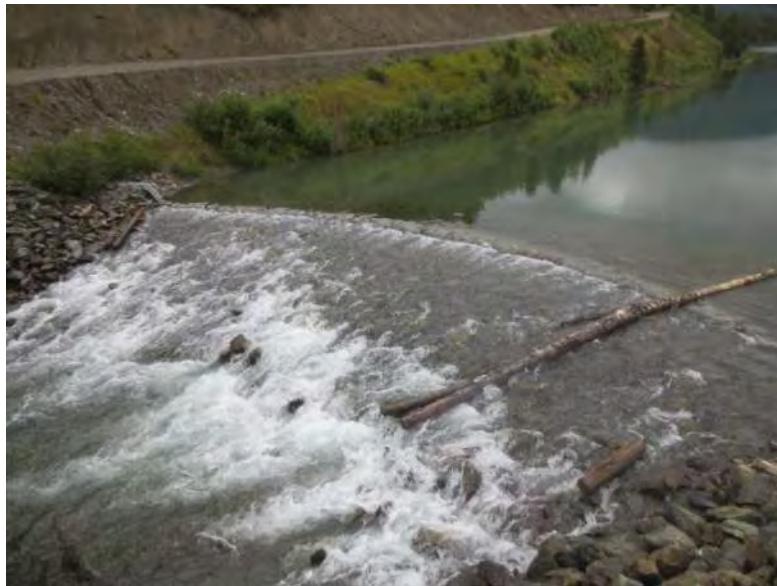
Photo 7: Existing weir at Surprise Lake
