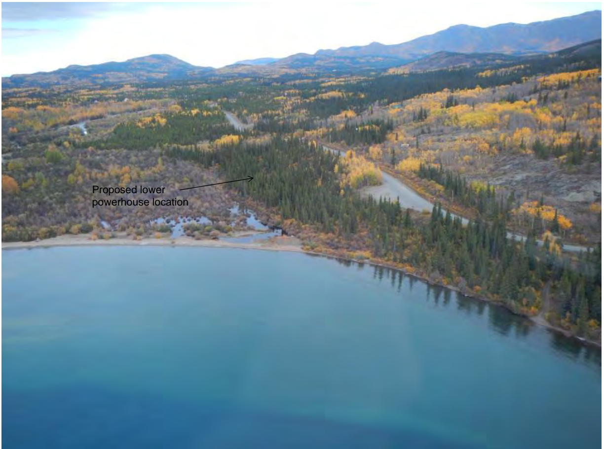
Photo 4: Proposed lower powerhouse location, looking east Proposed penstock alignment in background.
