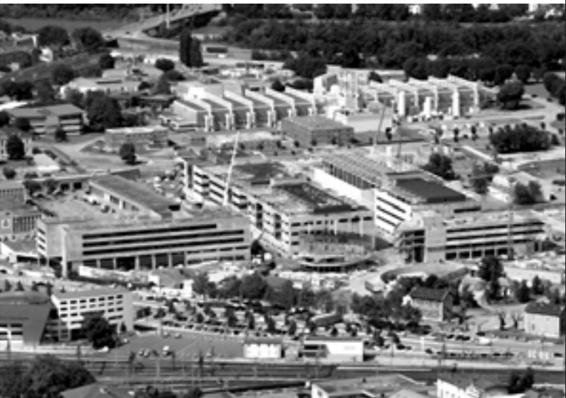
MINATEC - Under construction.
