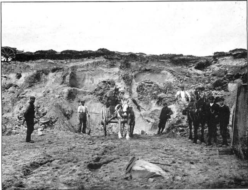
FIG. 1.—Leavad Sand Pit. General View.
